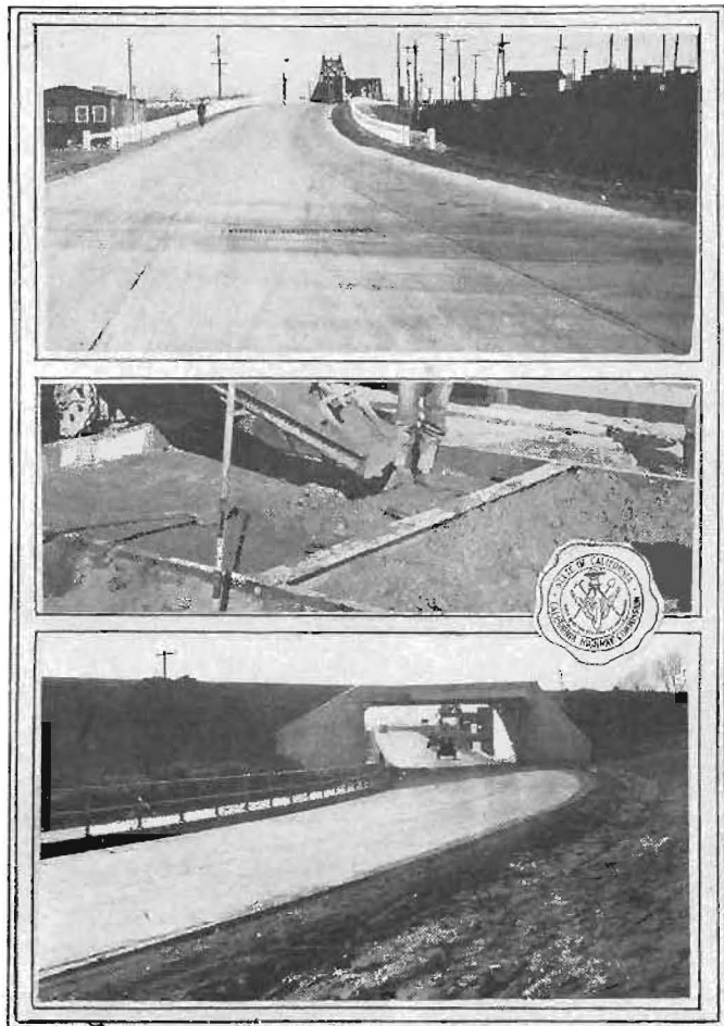
AT WEST SACRAMENTO—Above, new 30-foot pavement at approach to M street bridge; note center drain in pavement; center, method of holding transverse joints and dowels in place; below, new subway on improved alignment with safety walk for pedestrians.
