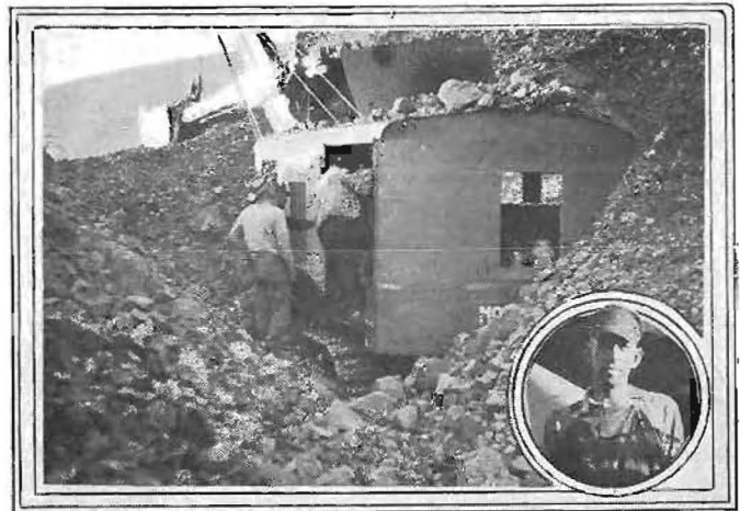
Shovel buried by slide while in operation near Point Mugu, Ventura County. Inset, Shovel Operator Dewey Alderson who risked life in effort to save equipment.
