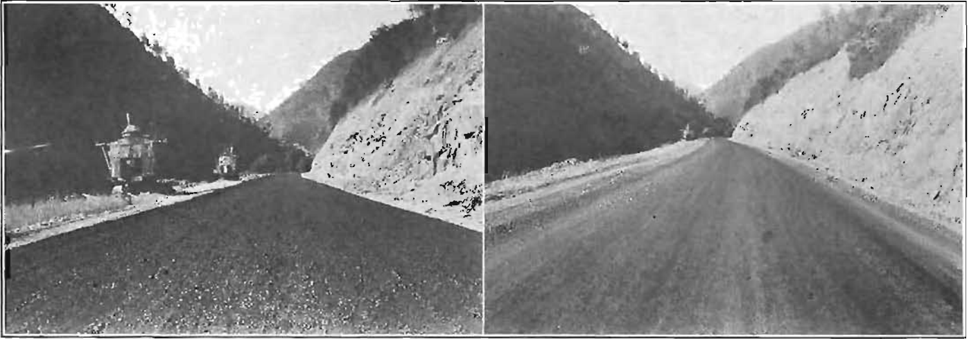
AFTER THE OILING TREATMENT.— Left , showing highways just after the oil process has been completed, but before opening to traffic; Right , shows the same highway compacted by several weeks of traffic.
