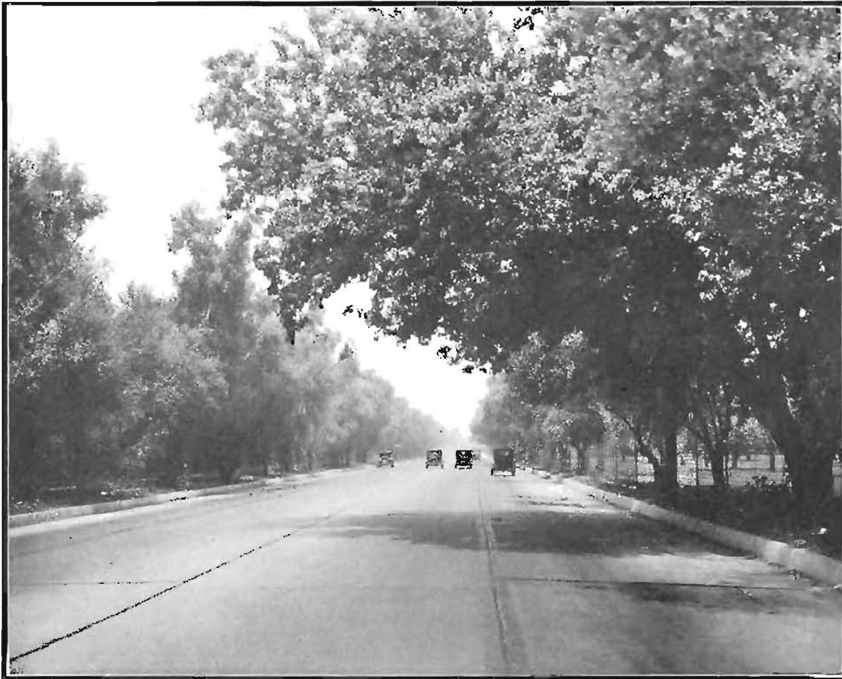
RESULTS OF COOPERATION.—Beautiful view of newly finished state highway near Whittier, the result of cooperation between Los Angeles County, a local road improvement district, and the California Highway Commission.
