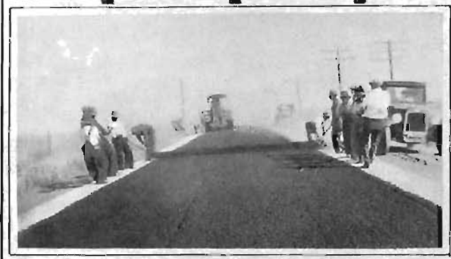
Upper, Rake used in mixing asphalt; Lower, Smoother surface obtained with strike-off templet.
