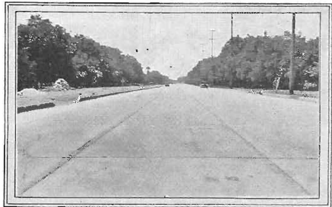
Ora-2-C: View of new 56' concrete pavement and curbs near Tustin, Orange County.
