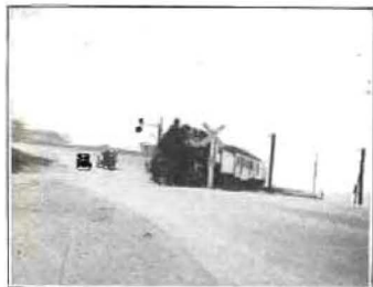
The old Del Mar grade crossing in San Diego County was a menace to the traveling public.
