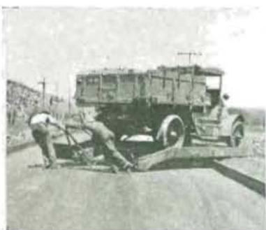
Turning a truck upon a road turntable.
