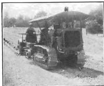
Step One— Heavy scarification
