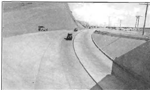
Another view of south subway.
