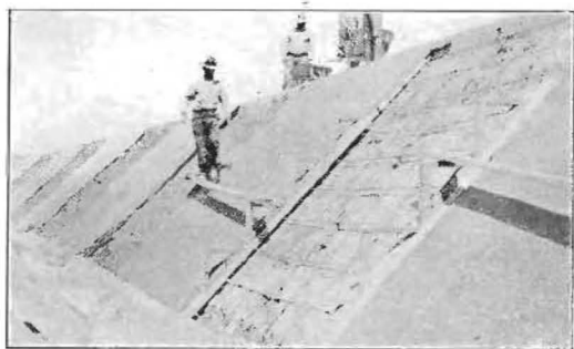
Placing slope paving in north subway.
