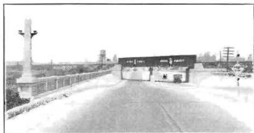
Undergrade crossing on state highway near Whittier in Los Angeles County consisting of two 30-foot roadways.
