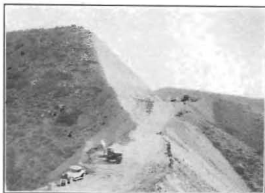
A cut and fill on Cajon Pass.
