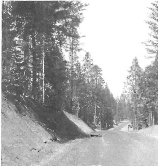
A highway slope cleared of inflammable material.
