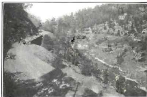
Scene on the Feather River lateral above the new bridge. This portion of the highway was built by convict labor.
