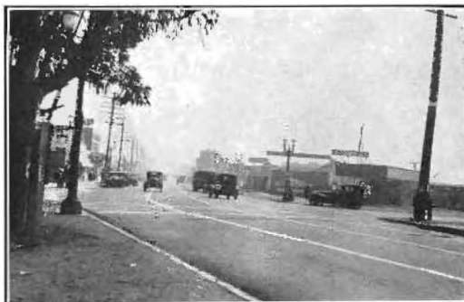
Traffic lanes leading into a California city.
