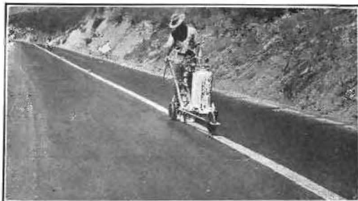
How the highway stripe is made.
