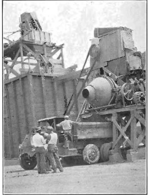
Mixing slurry base in drum mixer.
