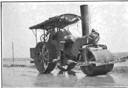
Rolling slurry base with macadam roller.
