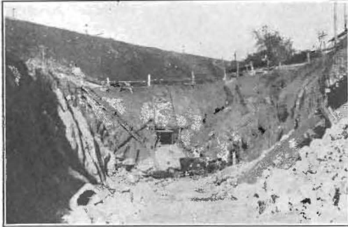
West portal of tunnel under Newcastle
