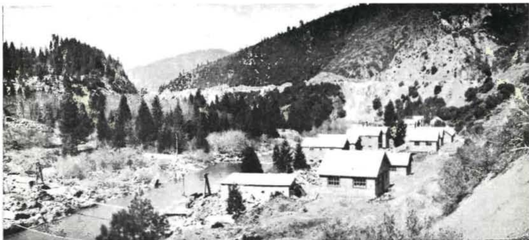
IN A SCENIC PARADISE, the labor camp for unemployed at Rich is located on the banks of the Feather River. Opened and maintained by the Department of Public Works, the men have comfortable quarters in substantial, heated two-story bunk houses close to their highway work.
