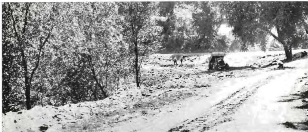
SURE TO PLEASE motorists, is this minor improvement on the State highway near Deadman's Springs, Amador County, where a sharp open curve was flattened out for safer driving.
