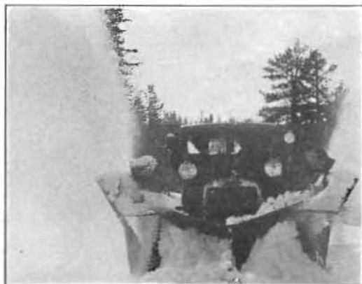
Dual motored four-wheel-drive truck with rotary plow, Donner Summit, 1930-31.
