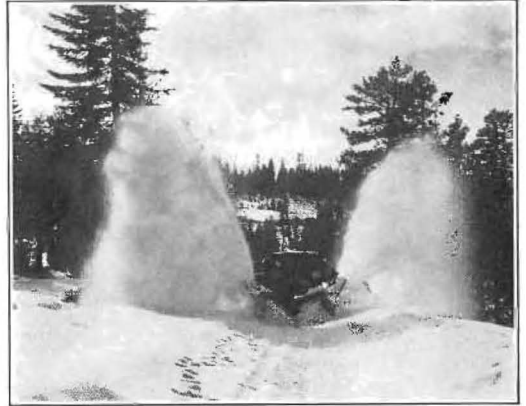
Rotary plow on dual motored four-wheel-drive truck, making first cut through two feet of snow, west of Soda Springs.
