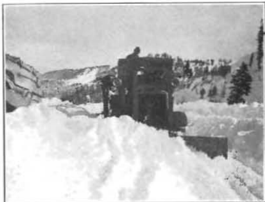
Push plow on three-ton, four-wheel-drive truck, clearing roadway on Donner grade, February, 1931.
