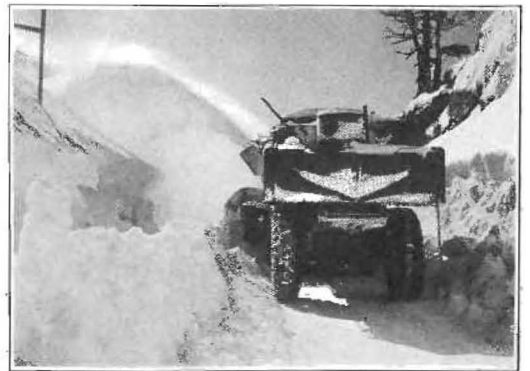
Rotary plow on four-wheel-drive truck, widening roadway through cut on Donner Summit, February, 1931.
