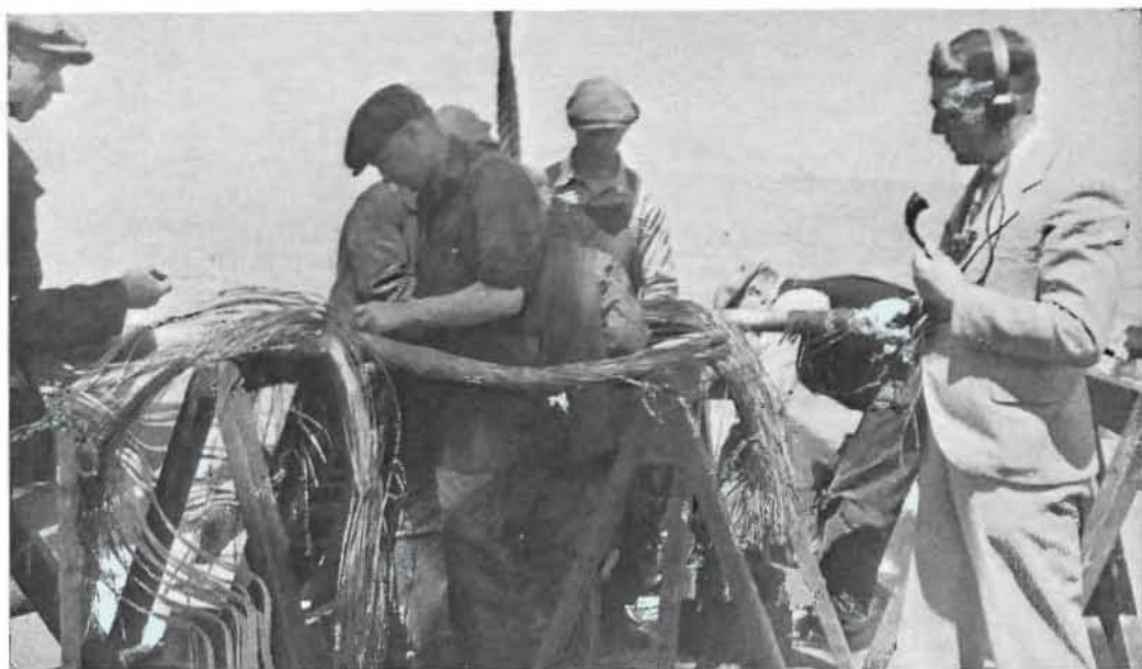
QUICK SERVICE —The Telephone Company putting finishing touches to a big job of moving phone cables out of the way of the Bay Bridge. At top, Diver William Reed (see the top of his helmet in the water) receiving telephoned instructions from Construction Superintendent F. O. Edmunds on the barge. And below, Edmunds has hooked up on a cable being spliced, to talk with headquarters ashore from the middle of San Francisco Bay.
