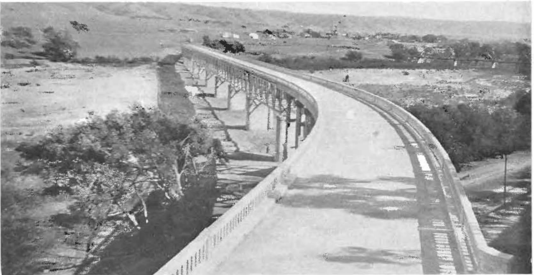
PERENNIAL YOUTH seems assured for this new concrete structure at Bradley by novel features that will permit the easy widening of its 24-foot roadway to meet future traffic conditions on the busy Coast Highway.
