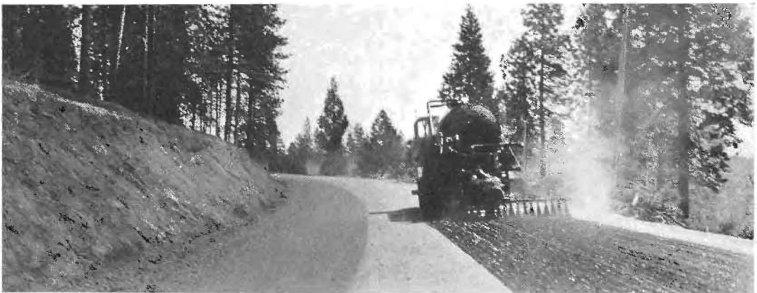
PAINTING THE ROAD with a thick coat of asphaltic oil this spreader truck swiftly lays a dustless surface where the old emigrant trains trundled for miles through murky clouds of powdered dirt.
