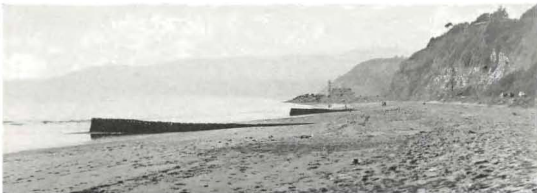
HARNESSING OLD OCEAN , compelling it to work in building up beach by use of groynes or bulkheads, this view shows results obtained on Santa Monica coast. Note tops of groynes nearly submerged by newly deposited sand.
