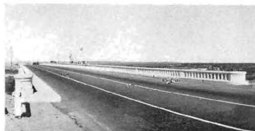
MODERNIZED by a widening operation and new concrete railings, the recently remodeled structure now provides a 46-foot roadway with sidewalk.
