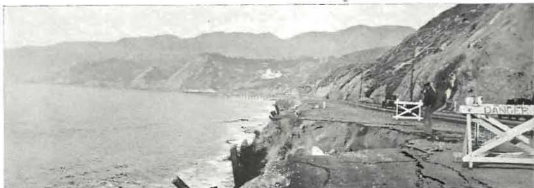
CONQUEST OF THE WAVES , soon to be ended, is depicted in this scene. Battering seas have wiped away the beach and are gouging out the highway slopes on this section of the Coast Boulevard northwest of Santa Monica.
