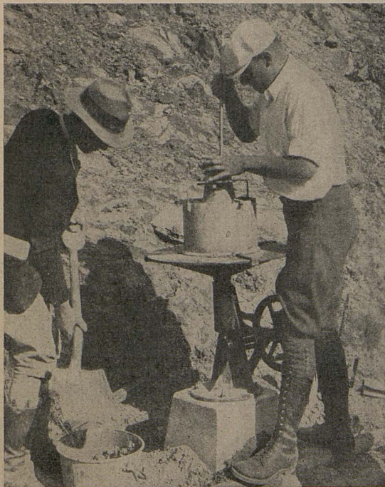
Making workability tests during construction
