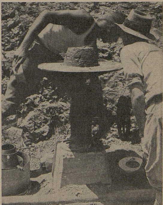
Flow test for determining concrete consistency
