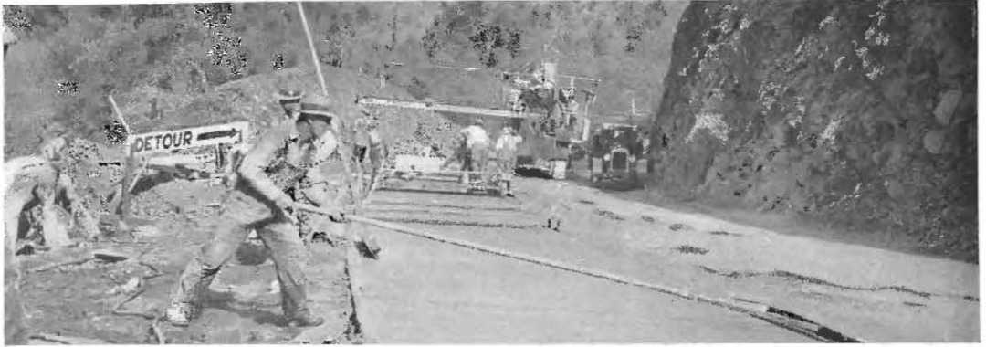
FAST WORK in finishing this new portland cement concrete paving job in Placer County was made possible by several devices created by State Highway engineers.
