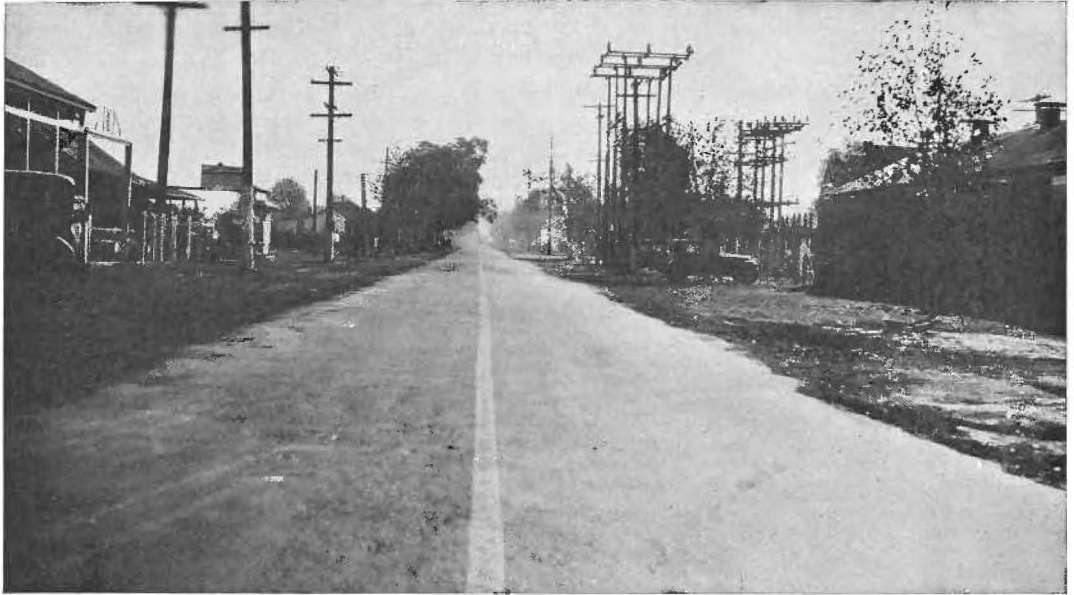
BEFORE cooperation came to Lodi in highway building in which State and city share the expense, this is how the State highway looked at the point where this main arterial known as Stockton Boulevard crosses the railroad tracks entering the city from the south.
