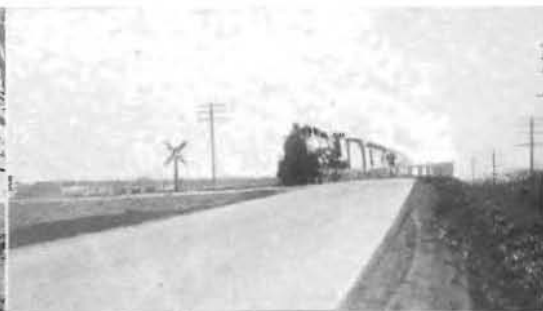
BAD SPOT , this was, where highway crossed the tracks at a severe skew, impairing visibility, augmenting danger.
