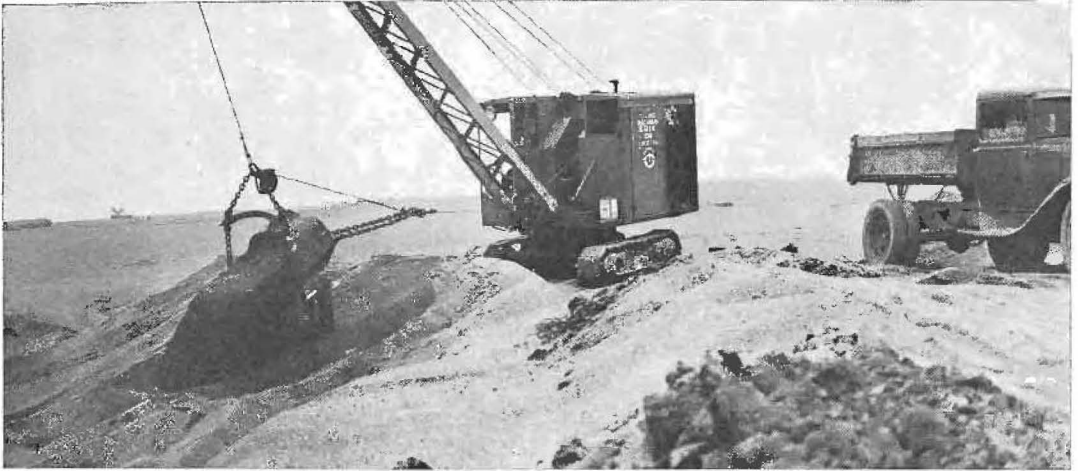
BEACH GOLD MINE this proved to be for the highway builders in Humboldt County. With no supply of aggregate available they tried beach sand for asphalt paving and it worked.
