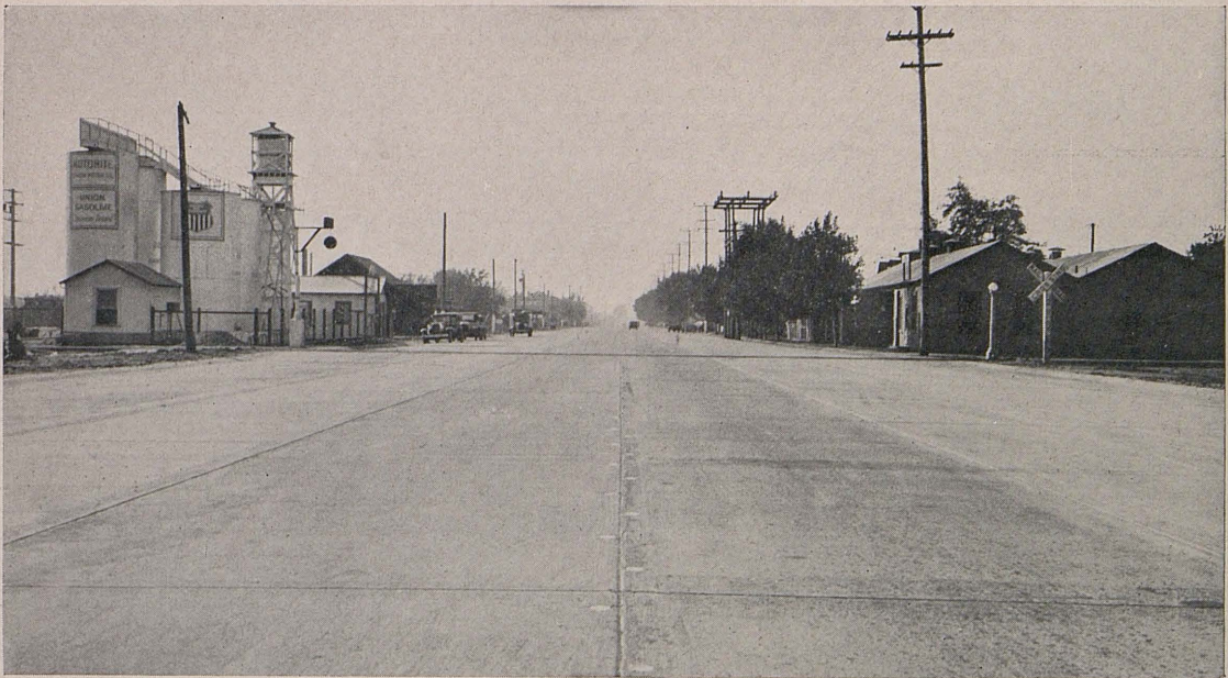
PORTLAND CEMENT CONCRETE pavement on Golden State Highway through Lodi in San Joaquin County.
