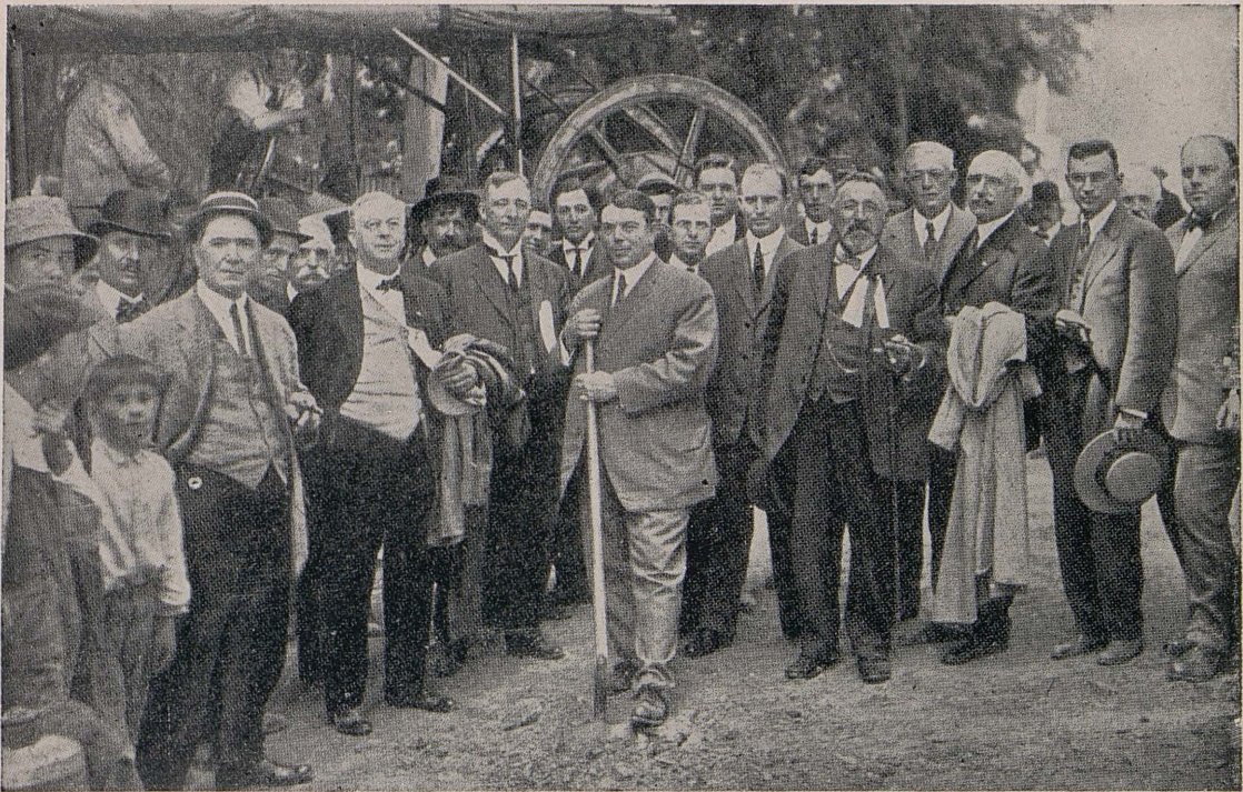
TWENTY YEARS AGO on August 7, 1912. Chairman Burton A. Towne of the first California Highway Commission turned the first shovelful of earth on the first State highway contract. The scene is reproduced from the book "California Highways" by Ben Blow, field secretary of the National Automobile Club.
