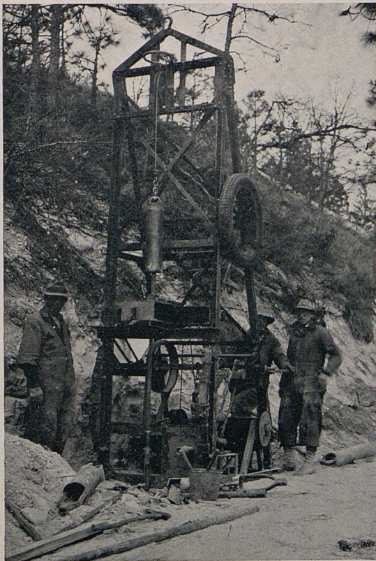
ON THE JOB , the trailer, up-ended operates as drill, sand pump or 200 pound trip-hammer hoist.
