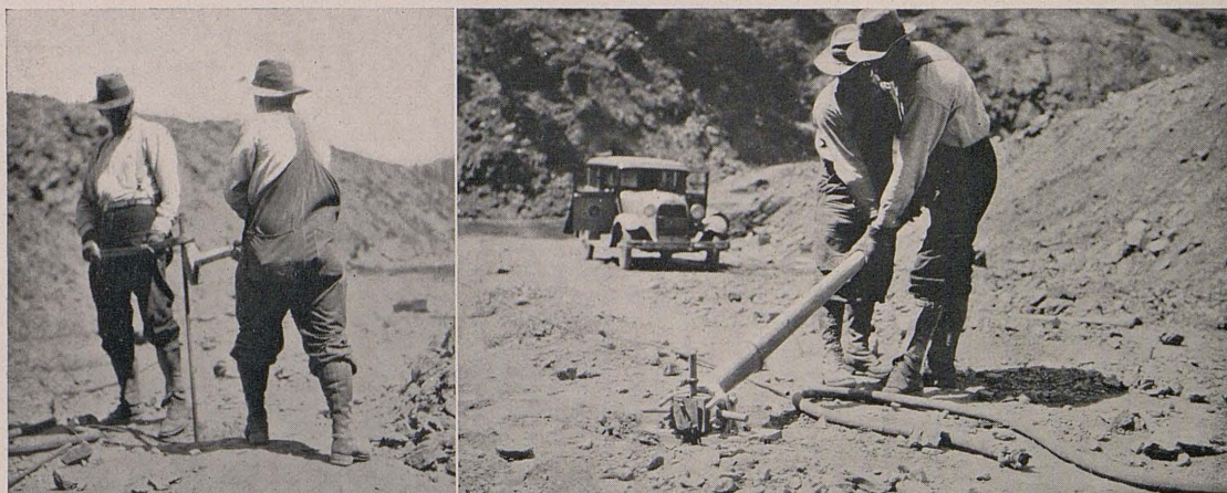
OLD AND NEW methods of extracting drill steel stuck in the hole are shown above. The old, lengthy and laborious sledge-hammer method has been eliminated by the Jumbo steel puller invented by Camp Superintendent Edward Rawson.
