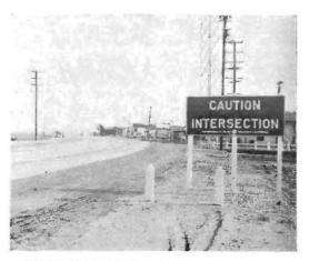
DAYLIGHT appearance of reflectorized warning sign showing method of erection.
