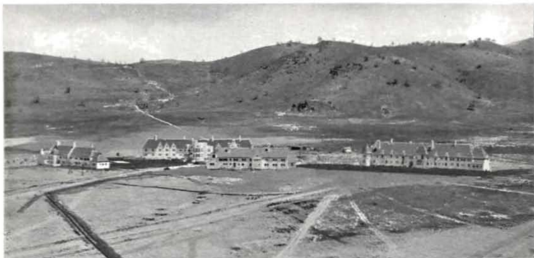
ART AND HEART went hand in hand in planning this group of buildings for the California Institution for Women, located in Cummings Valley near Tehachapi, Kern County. Housed in these spacious, well equipped structures of Norman architectural design, women heretofore crowded in San Quentin will be rehabilitated for their return to society. The large Detention Building and two dormitory cottages are at the left of the group with the Administration Building at right. This air-view was taken by the 115th Photo Section, Fortieth Division Aviation, California National Guard, Griffith Park, Los Angeles.
