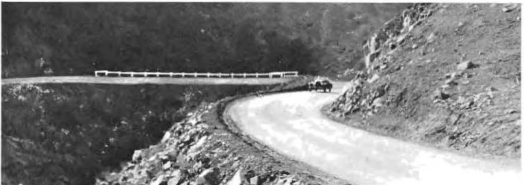
BEAUTIFUL BUT TOUGH for the highway builder are the many deep gulches that add scenic interest and numerous hairpin turns to this existing link on the All-Year route. They are avoided in the new location nearer the stream sources.
