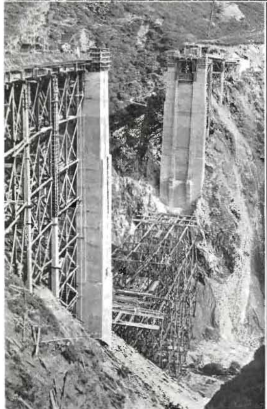
HIGH WIDE AND HANDSOME will be the 330-foot span made by the open spandrel deck concrete arch of the bridge across Bixby Creek on the Carmel-San Simeon coast highway. The above views show the record-breaking arch under construction.
