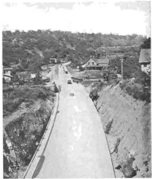
TIME AND MONEY saving to motorists are evidenced by this view from the East portal.
