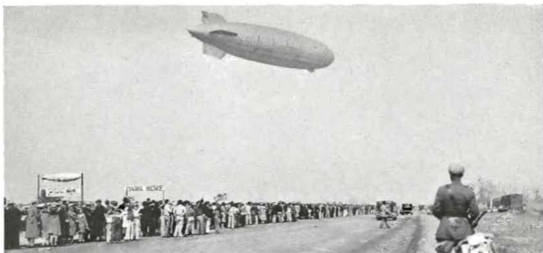
OUT OF THE MISTS of the morning the great U. S. Navy Dirigible Akron appeared above the newly completed link of the Bayshore Highway that passes the Air Base at Sunnyvale affording a vantage point for thousands of motorists and pedestrians who gathered in the early dawn to greet her.
