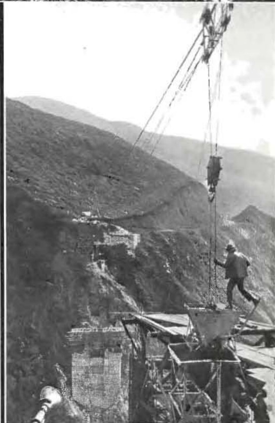
HIGH WIDE AND HANDSOME will be the 330-foot span made by the open spandrel deck concrete arch of the bridge across Bixby Creek on the Carmel-San Simeon coast highway. The above views show the record-breaking arch under construction.
