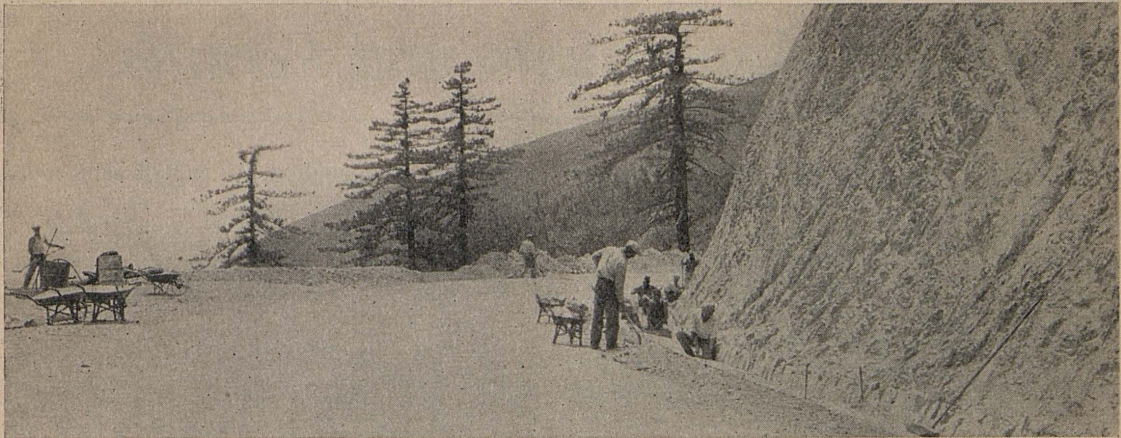
PROTECTION AND PREVENTION are exemplified in the above scene. Contingents of unemployment relief workers are building rock gutters to catch drainage waters from the mountain slope, thus protecting the road.
