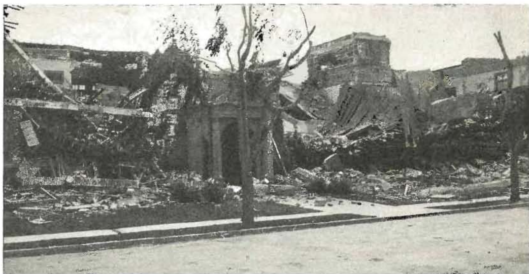
FAULTY CONSTRUCTION was responsible for the collapse of some school buildings in the recent earthquake area. A type of construction incapable of resisting horizontal earth movements is illustrated in the above picture. The State has stepped in to prevent the erection of such school buildings in the future by rigid control of design plans, specifications and inspection.
