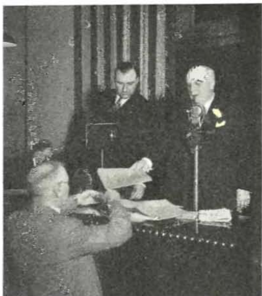
FIRST BID opened by Governor James Rolph, Jr., on a construction contract for the San Francisco-Oakland Bay Bridge is handed to Chief Engineer C. C. Purcell for tabulation while Director of Public Works Earl Lee Kelly assists at the proceeding.
