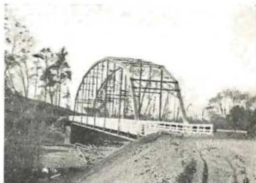
Practical economy is represented in this old Mad River Bridge moved to a new location, abolishing four railroad grade crossings.
