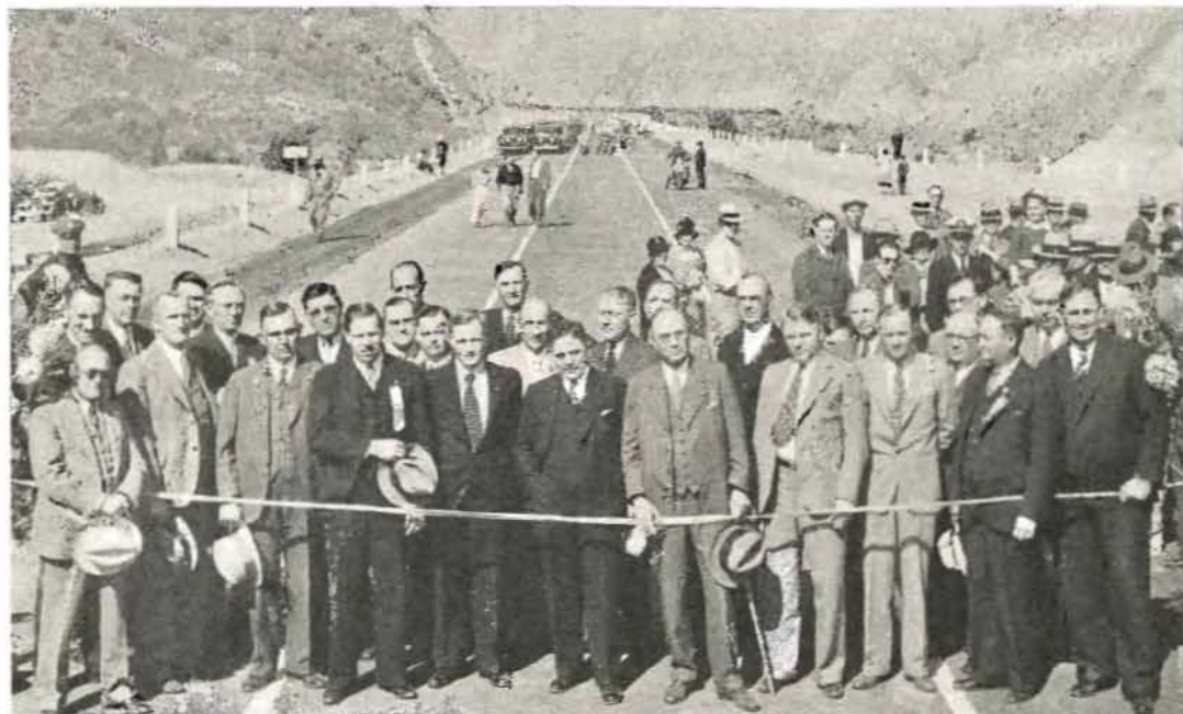
OFFICIAL GROUP at Ridge Alternate ceremonies: (left to right) Secretary Howe, Highway Commission; Asst. State Highway Engineer McCoy; Acting Dist. Engineer Gillis; Dist. Engineer Cortelyou; Asst. Resident Engineer Telford; Chief Engineer East Auto Club of So. Calif.; Supervisors Mitchell, Orange and Brite of Kern; Asst. Dep. Director Public Works Keaton; Contractor N. F. Jahn; Secretary Nourse, Kern Chamber of Commerce; Resident Engineer Templeton; Assemblyman Rogers, Los Angeles; Wm. Shoemaker, Orange; Col. A. Marks, Taft; Chairman Hopkins; C. C. Carlton, State Rights of Way Chief; Acting Dist. Const'n Engineer George; Highway Commissioner Stanton; Nat Neff, Orange County Engineer; President Louden, Economic Council, So. Calif.; Secretary Brashear, L. A. Chamber of Commerce; Carl Mock, Santa Ana Chamber; City Manager Nighbert, Bakersfield; Editor McCracken, Anaheim; Supervisor Wimmer, Kern County; President Simpson, L. A. Chamber of Commerce; Supervisor Quinn, Los Angeles County.
