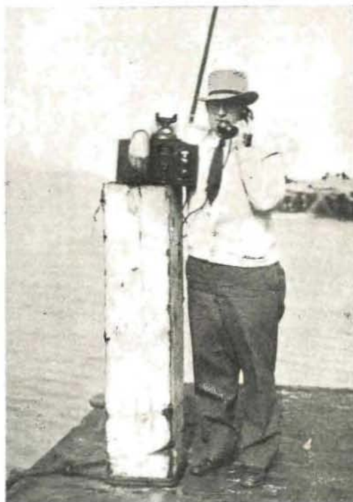
HELLO FROM BAY —Inventor D. Reginald Tibbetts speaking by radiotelephone from a work barge to the San Francisco-Oakland Bay Bridge offices in city.
