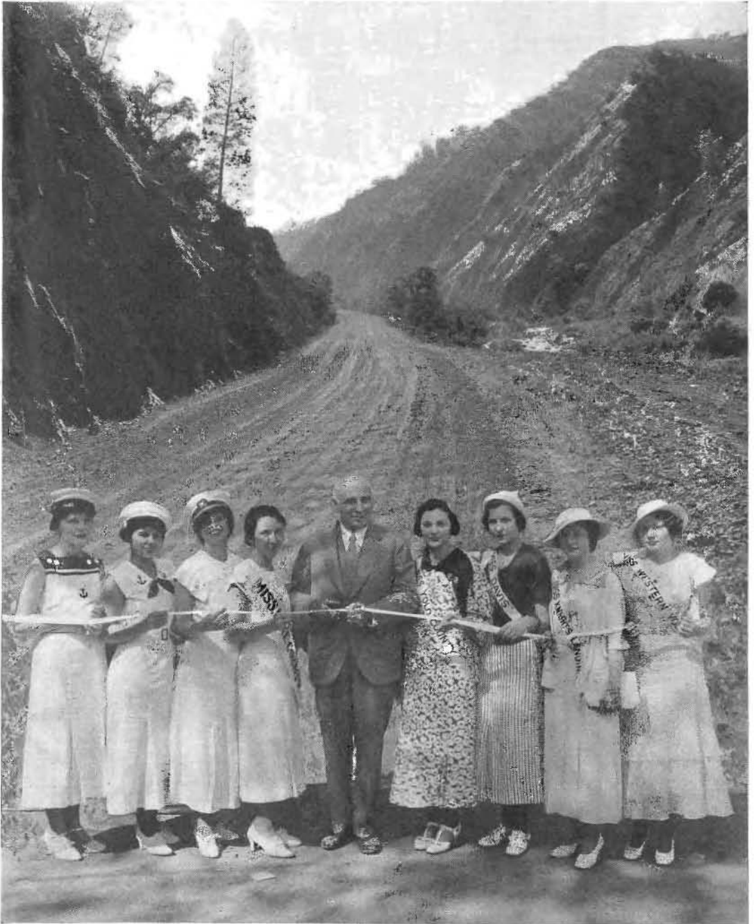
A REAL JUBILEE EVENT for the citizens of Yolo, Colusa and Lake counties occurred on August 4th when Governor Merriam officially opened and dedicated the new Rumsey-Clear Lake Highway affording a short cut through the mountains to the great recreational area of the Clear Lake region and the North Coast country. A portion of the scenic highway near Rumsey is shown above with Governor Merriam being assisted in the ribbon cutting by an octette of lovely girls of Yolo and Lake counties. At the left are three Clear Lake yachting girls led by "Queen" Vera Behrens of Kelseyville. At the right is "Queen" Wanda McGrew of Woodland representing Yolo County accompanied by Miss Davis, Miss Knights Landing and Miss Western Yolo County. After the ceremony a caravan of autos traversed the 15 miles of new road into Lake County.
