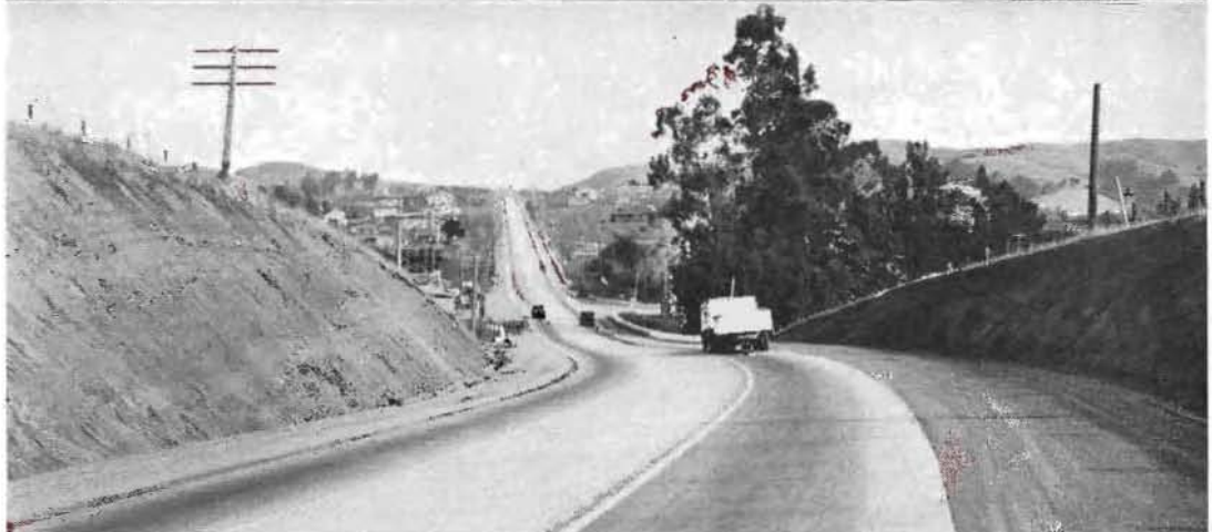
STRAIGHT THROUGH THE HILLS runs the new, shorter Dublin Canyon Boulevard on a high standard of alignment with a minimum of curves and a maximum of sight distance and 6 per cent grade. No. 1—General view of three-lane highway through central part of canyon showing elimination of many curves. Nos. 2 and 3—Comparative views of new and old highway taken at same location. Below—The broad curve on Castro Hill with three lanes widening to four-lane 40-foot pavement.
