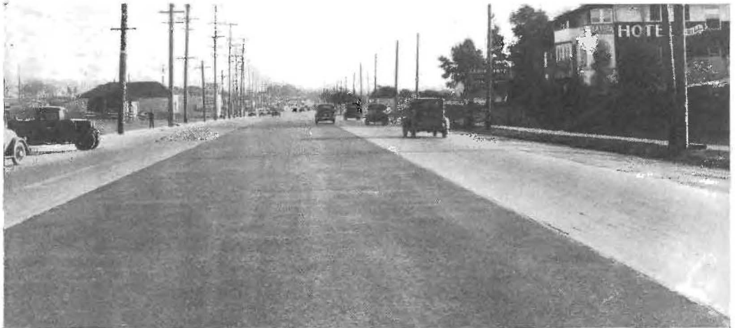
FINISHED PRODUCT presents a 74-foot pavement adding two broad lanes for motor vehicle traffic.
