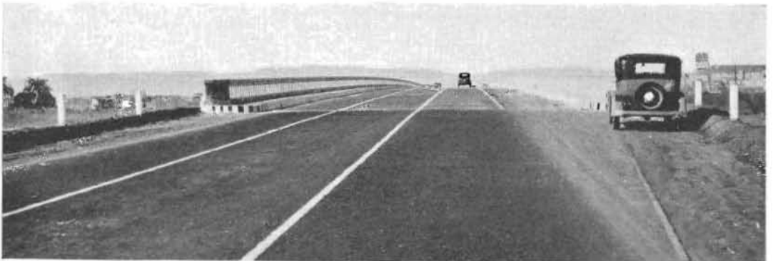
OVER THE SAN DIEGO RIVER, a noble steel and concrete bridge carries the new highway on a 40-foot roadway. It has a total length of 641 feet.
