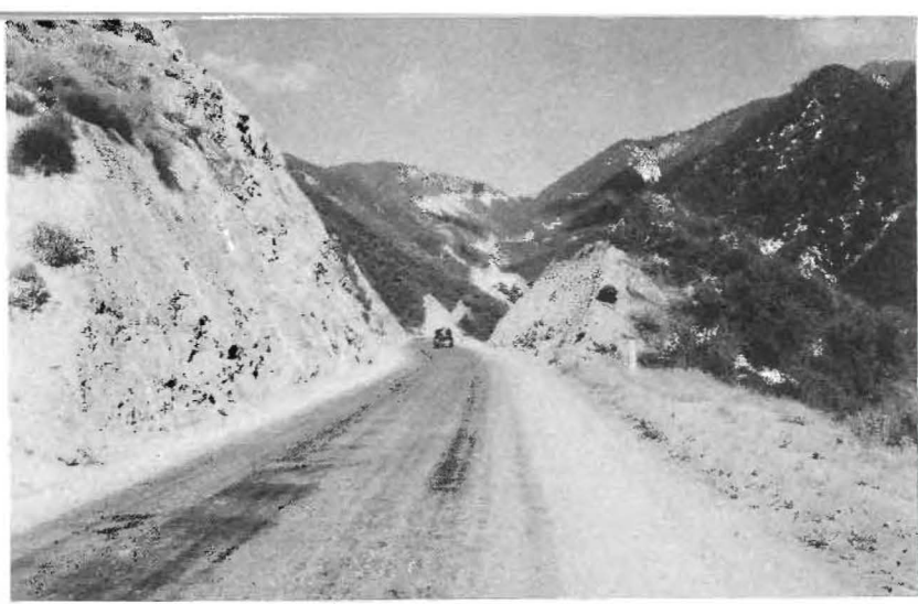
GRADING OPERATIONS call for 914,000 cubic yards of roadway excavation, 5,000,000 yards overhaul.
