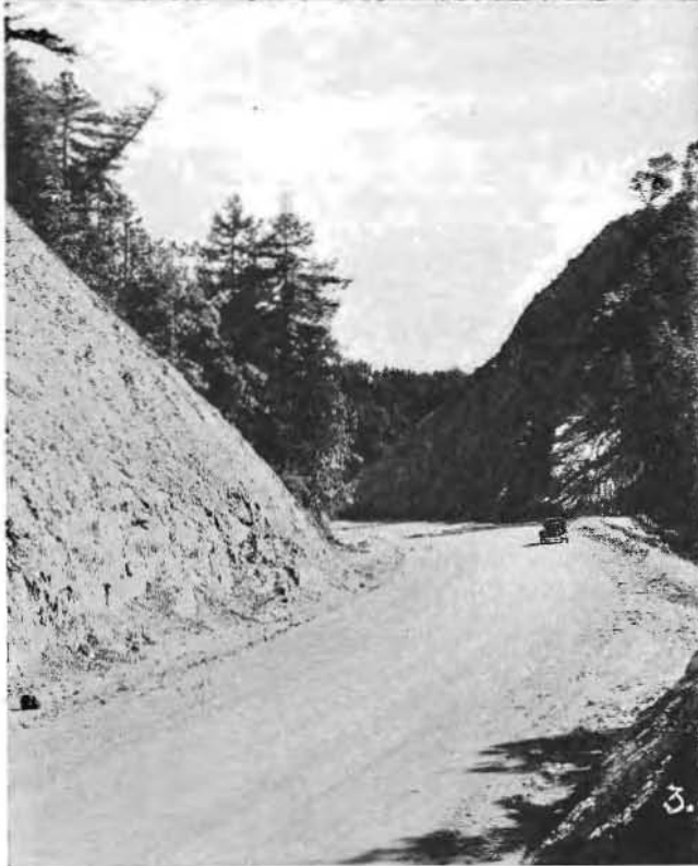
OVER THE MOUNTAINS between Los Gatos and Santa Cruz a fine new highway link is approaching completion, replacing a narrow old road of poor alignment. Parts of the new Scotts Valley-Inspiration Point link that cuts out 130 curves on State Route No. 5 are shown above. No. 1—Old and new road entering north city limits of Santa Cruz. No. 2—A view of the new road at Inspiration Point, showing a bit of the old route winding down around a cliff at the left. Nos. 3 and 4—Two of the deep cuts through the hills.
