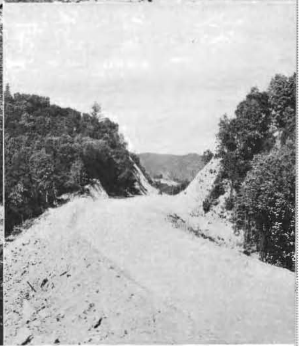
OVER THE MOUNTAINS between Los Gatos and Santa Cruz a fine new highway link is approaching completion, replacing a narrow old road of poor alignment. Parts of the new Scotts Valley-Inspiration Point link that cuts out 130 curves on State Route No. 5 are shown above. No. 1—Old and new road entering north city limits of Santa Cruz. No. 2—A view of the new road at Inspiration Point, showing a bit of the old route winding down around a cliff at the left. Nos. 3 and 4—Two of the deep cuts through the hills.
