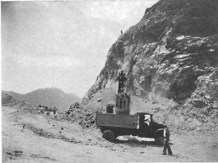
WIDENING OPERATIONS call for heavy work on mountain spurs encroaching on the alignment.
