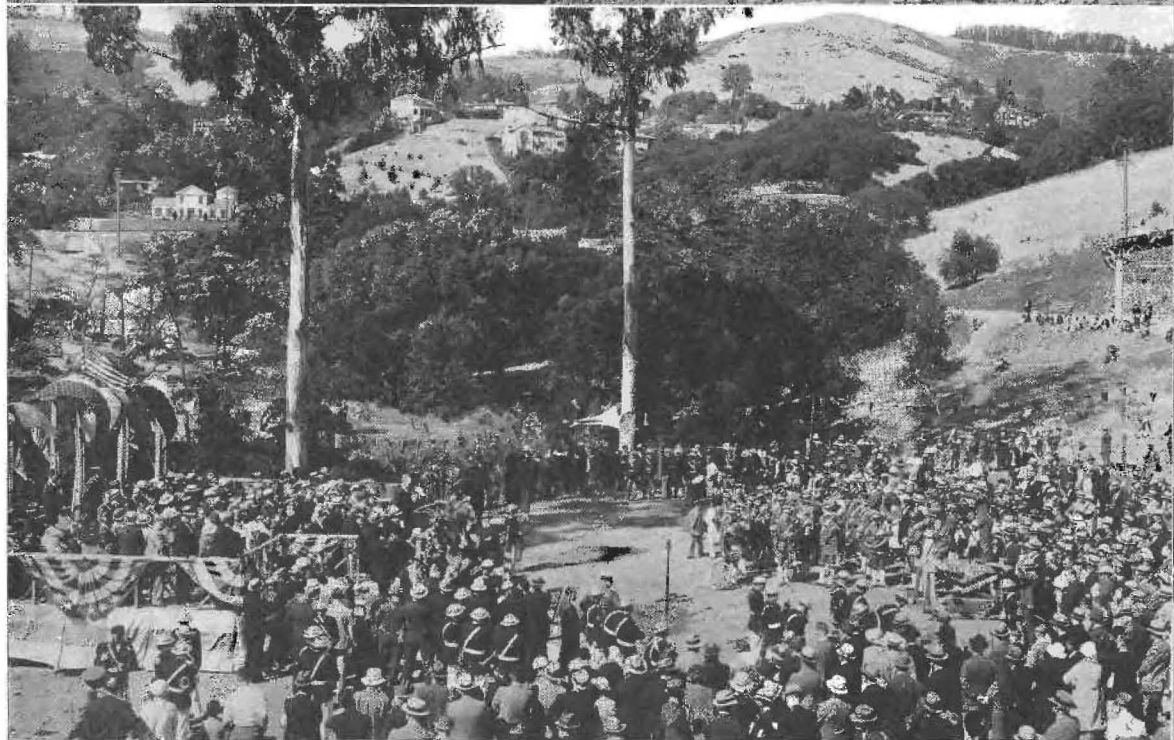
STARTING WORK ON A GREAT PROJECT, Governor Merriam and Director Earl Lee Kelly participated on June 17 in ground breaking ceremonies at Oakland for the Broadway low level tunnel to connect Alameda and Contra Costa counties. In the upper picture Governor Merriam is seen turning the first shovelful of earth assisted by Director Kelly; Supervisor T. E. Caldecott, chairman of Joint Highway District No. 13; Dudley W. Frost (kneeling), chairman of Oakland and Berkeley Junior Chamber of Commerce Committee, and a group of young women representing participating communities. A beautiful eucalyptus grove at Broadway and Chabot Road, Oakland, was the scene of the formal exercises, which included speechmaking, music of massed bands, pageantry and fireworks.
