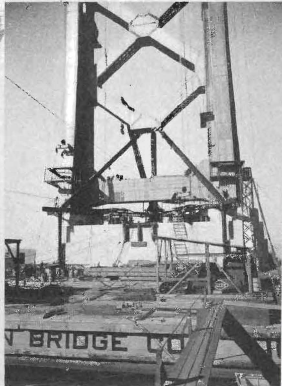
RISING SKYWARD above the city's shoreline, Tower W-2 of the San Francisco-Oakland Bay Bridge presents fascinating studies of majestic beauty and strength to the camera. A side view shows the slender, graceful silhouette tapering from the base to its top 474.35 feet above the water. A worm's eye view presents a vaulting pyramid of steel lattice work. Seen through a second story office window it dominates all the bay front structures, its top almost lost in the cloud vapors. A close-up reveals the massive size of the great steel girders.
