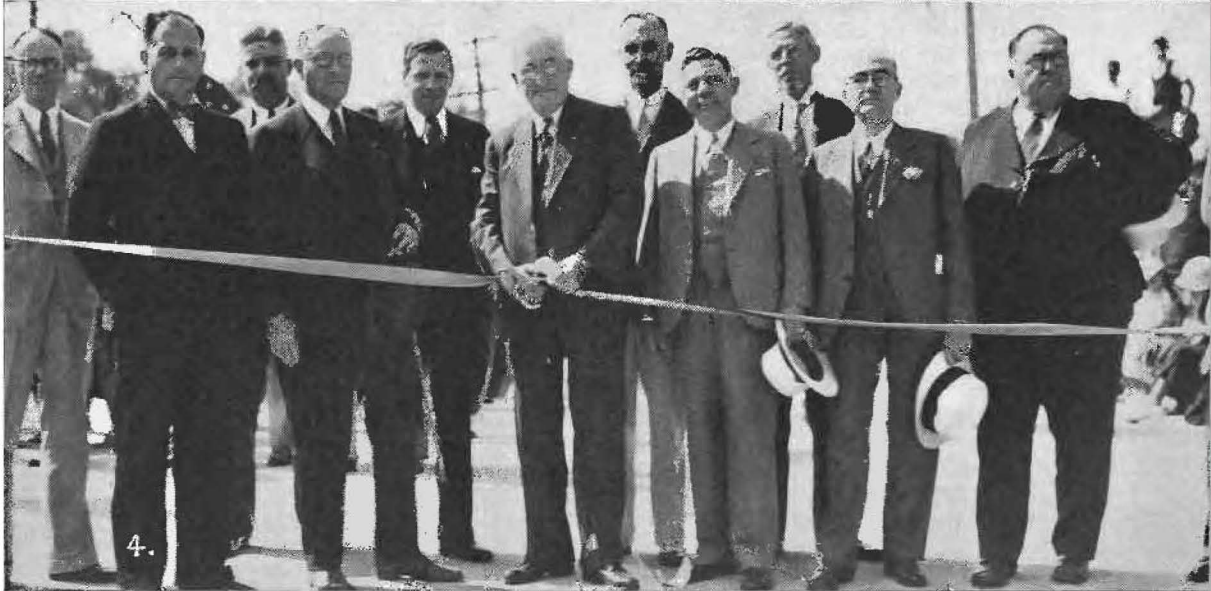
A BROAD SPAN of concrete and steel now carries the highway over the railroad yard at San Bernardino as shown at top. 2. One of the wide, flaring approaches. 3. Old, narrow structure with right-angle turn. 4. Official group at dedicatory ceremonies (left to right): Chamber of Commerce President Ray Stockwell; Mayor A. W. Seccombe; State Bridge Engineer F. W. Panhorst; Highway Commissioner P. A. Stanton; Deputy Director of Public Works Morgan Keaton; Highway Commissioner F. A. Tetley; Chairman C. C. Whitney; Harry A. Hopkins, Chairman Highway Commission; Mayor E. F. Harford, Colton; R. H. Mack, Secretary Chamber of Commerce; Supervisor John Andreson.
