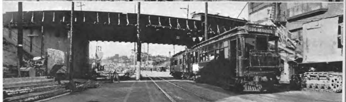
BUSY SCENE IN CITY'S HEART. Activities attendant upon the construction by the State of the $130,000 viaduct now being built over Glendale Boulevard at the intersection with Sunset Boulevard in the city of Los Angeles is shown in the top sketch by Artist Charles Owens of the "Los Angeles Times." The lower photographs show how the excavation and building work is being carried on without interrupting traffic of the two street railway lines on both levels of the grade separation.
