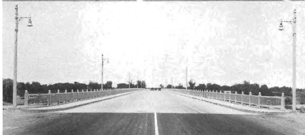
BAKERSFIELD BY-PASS UNITS examples of modern construction. At top, four-lane steel and concrete overpass spanning railroad tracks. Center, portion of 30-ft. asphaltic concrete pavement with 3-ft. shoulders. Below, steel and concrete bridge over Kern River, 2293 feet long with 40-ft. roadway.
