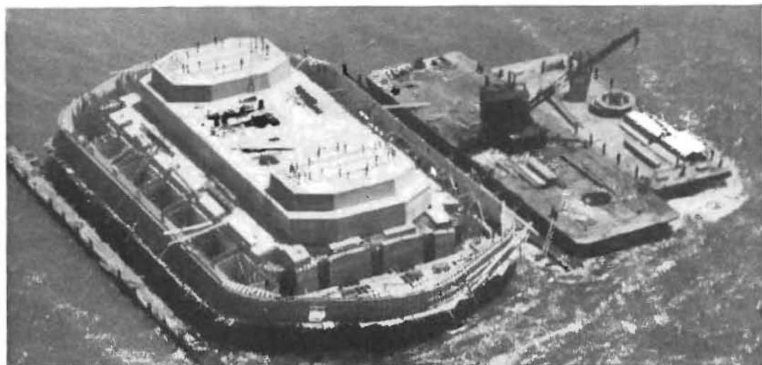
ANOTHER WORLD'S RECORD is represented by Pier W-6 of the Bay Bridge, located 1160 feet west of Yerba Buena Island; the first pier ever built and completed by the compressed-air-flotation caisson method.
