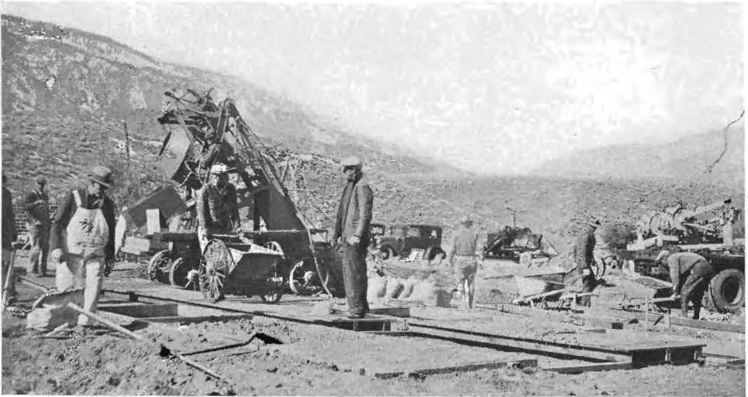
A PAVING EXPERIMENT is here pictured as conducted on the Ridge Route Alternate last winter. Fourteen test sections of cement concrete were cured under different temperature conditions.
