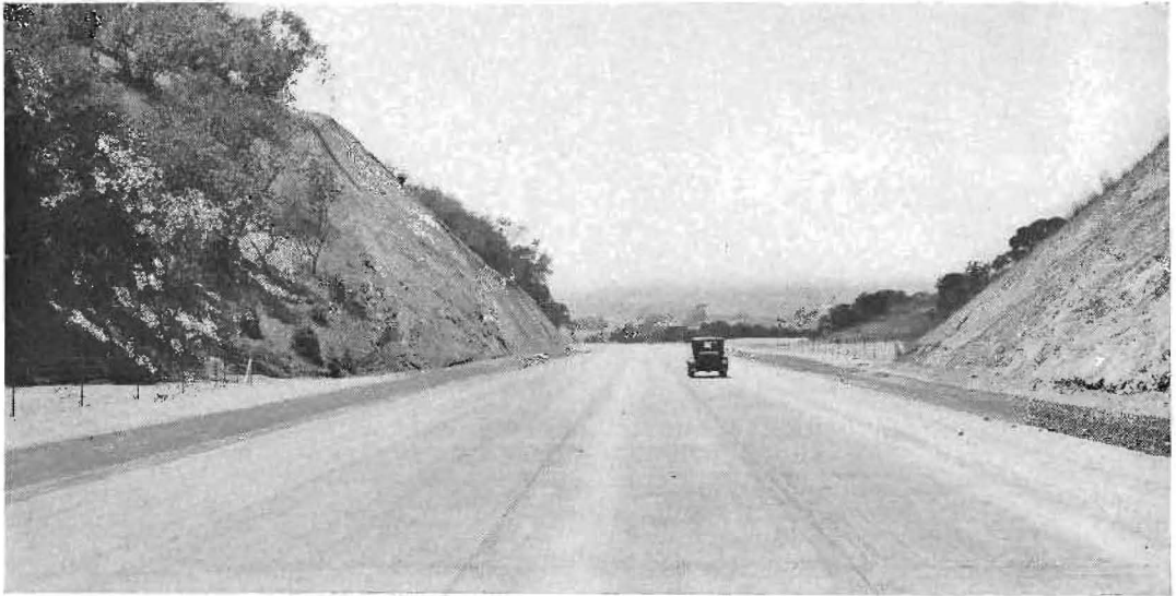
MANY BIG CUTS on Los Angeles-Pomona Highway permit a direct route through hills and wide oiled shoulders give additional width to broad traffic lanes.
