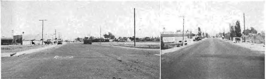
BEFORE AND AFTER views of the improved link of State highway through the city of Anaheim. At left is the newly paved and widened North Los Angeles Street, now a fine broad thoroughfare. At right is the old street narrowed by encroachments and obstructions.
