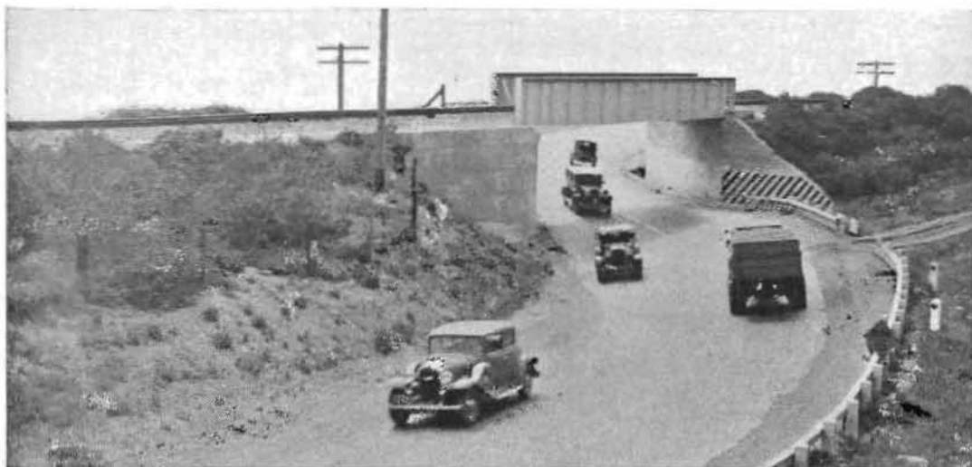
OBSOLETE UNDERPASS , of narrow width and poor visibility that will be eliminated by realignment of the Coast Route north of Ventura.
