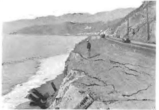
OLD OCEAN HARNESSSED by groins has been toiling for State highway engineers building a fine sandy beach along the Santa Monica Coast where no beach existed. In 20 months it has made a beach a mile long and 200 feet wide as shown by shaded portions of the drawing by Artist Phil Leonard of the Los Angeles Times. It provides a public bathing beach as well as a protection to the highway. Photo shows how the waves were gouging out the highway shoulders before groins were installed.
