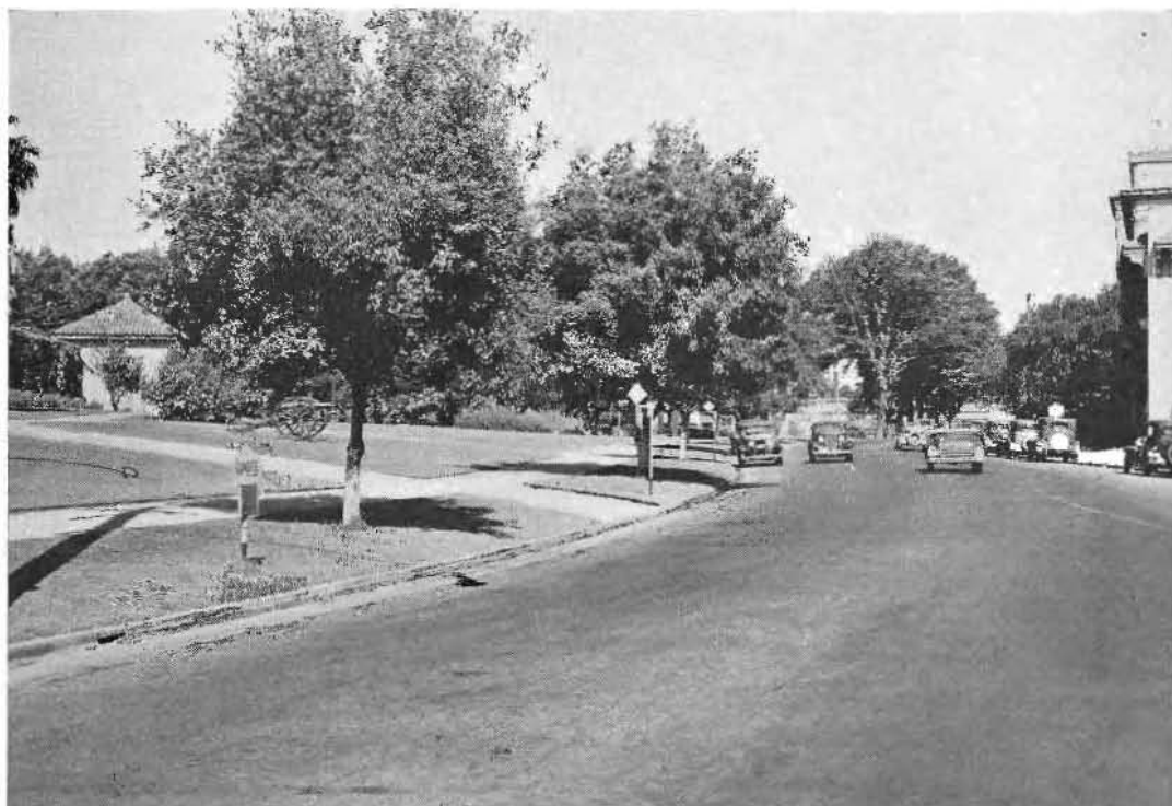
GAS TAX PAVEMENT recently completed on "L" Street in the city of Sacramento where State Highway Route No. 4 passes the historic Fort Sutter situated in Sutter Park.
