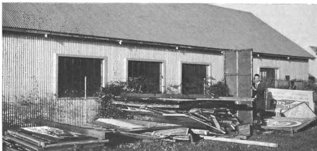
STORAGE PILES ARE GROWING —Structures removed are carefully stored in various highway maintenance yards awaiting reclamation by owners.
