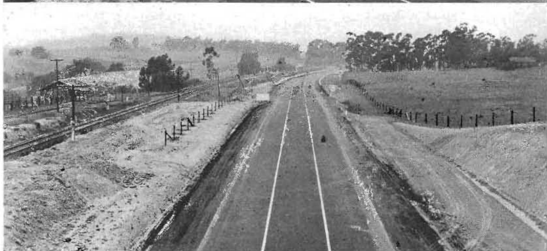
THROUGH TRAFFIC BOULEVARD recently completed in the city of Santa Barbara is a 3-lane, asphalt concrete highway 5.9 miles relieving the city's congested district of much heavy Coast Route traffic. The upper picture shows a section extending from Carillo Boulevard near the easterly city limits. The Mission Creek bridge sector is seen in the center photo and below a portion of the westerly unit leading to the intersection with the Coast route at Central Avenue.
