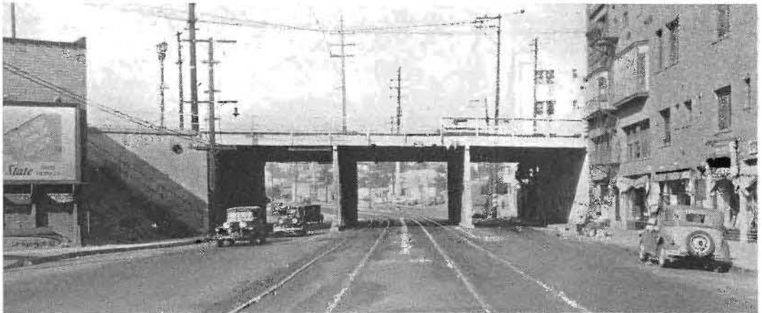
RELIC OF EARLY CONSTRUCTION standards this old timber bridge has been replaced by the new concrete and steel viaduct. Besides being inadequate to carry the load of present day traffic, its heavy wooden supports obstructing the roadway were a menace to vehicles.
