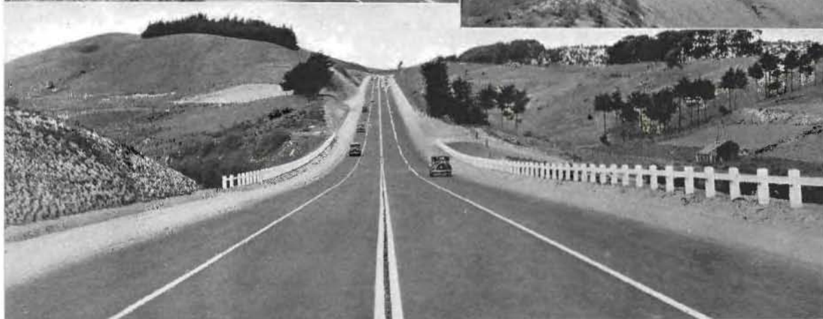
LATEST MODERN STANDARDS of highway construction are incorporated in the recently completed extension of Junipero Serra Boulevard, one of San Francisco's main arterials down the Peninsula. The new unit, 1.67 miles long, is graded to a width of 65 feet including a small berm on hills. The 40-foot pavement is 6-inch asphalt concrete on 4-inch crusher run base. The shoulders of 4-inch crusher run base have an oil bound surface and shoulder treatment is extended to adjacent gutters. Maximum grade is 5 per cent. Double striping marks the center of the four traffic lanes.
