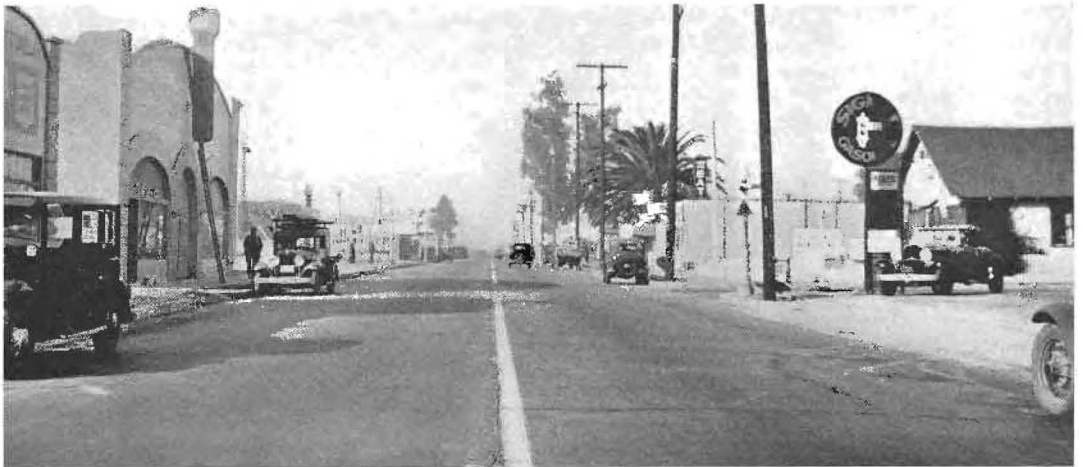
OLD BOTTLENECK CONDITION as it existed before the improvement is shown above. The old pavement was only 40 feet wide, much too narrow for the heavy traffic on this route. The section recently completed is 1.49 miles in length and has a right of way with 100 feet for the entire distance.
