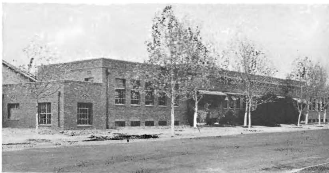
GROWING WINGS the Testing and Research Laboratory of the Division of Highways at 34th and Serra Way is expanding to take care of increased work. The wings add 5000 square feet of floor space.
