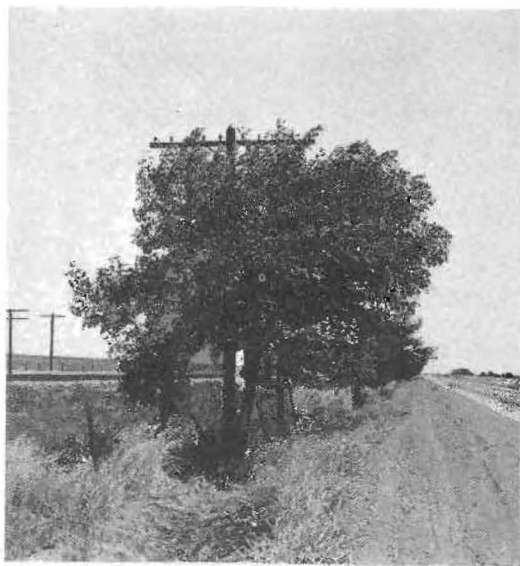
AT CLOSE QUARTERS, with wires above tree growth, poles must be raised.
