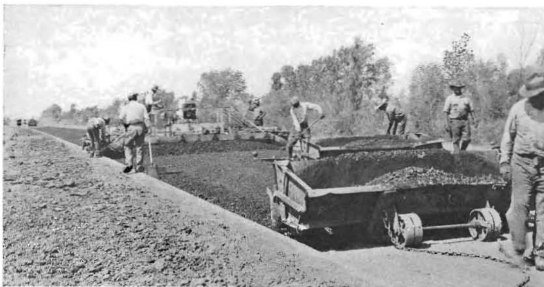
PLACING ASPHALT CONCRETE BASE COURSE on contract in Sacramento County.
