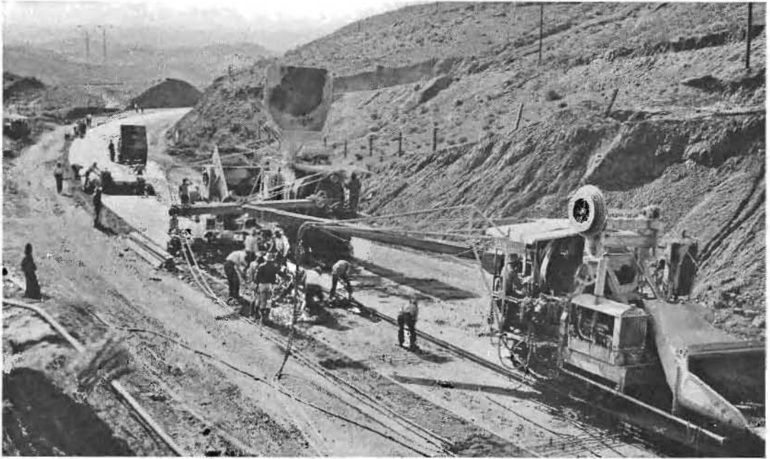
TWO PAVERS laying Portland cement concrete on Ridge Route alternate.
