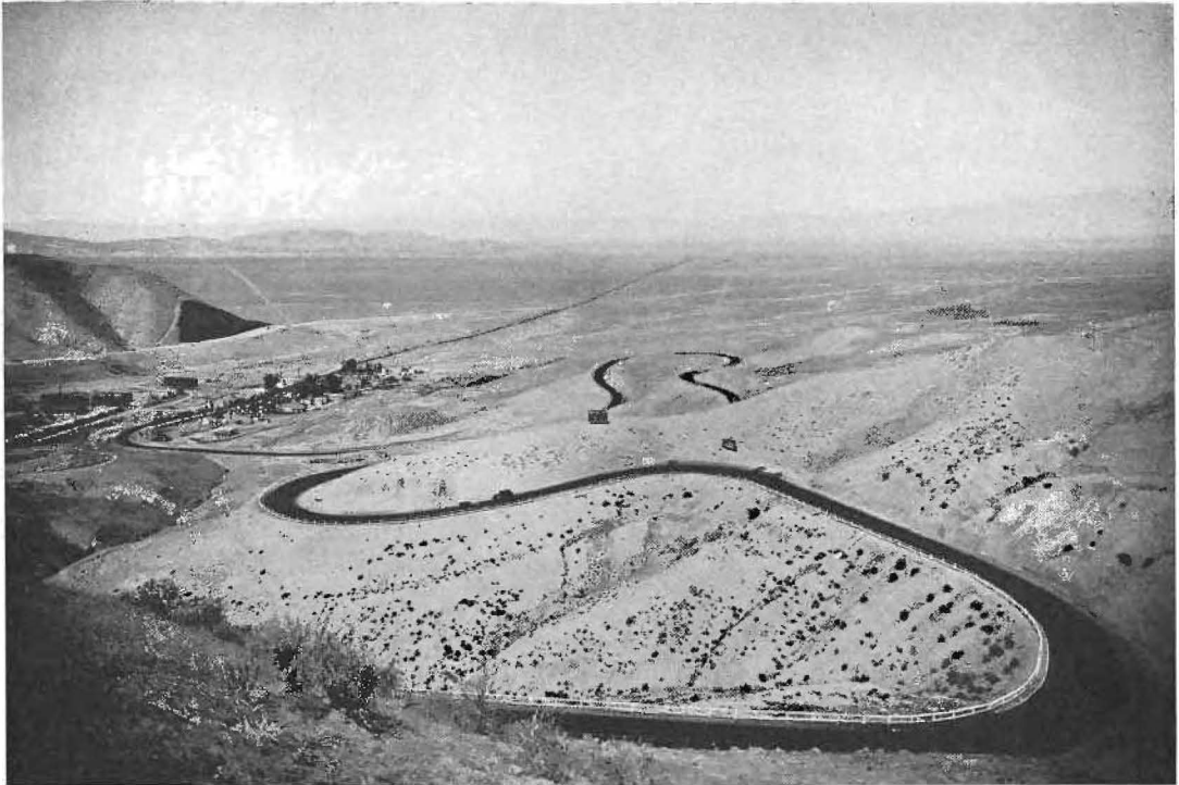
A SINUOUS COURSE with many sharp turns is followed by the existing Grapevine Grade sector of old State highway between Fort Tejon and Grapevine Station on the Los Angeles-Bakersfield arterial. The new alignment soon to be opened is shown at the extreme left center passing a huge slope cut of the high hill and joining the present straightaway to Bakersfield a mile to the north.
