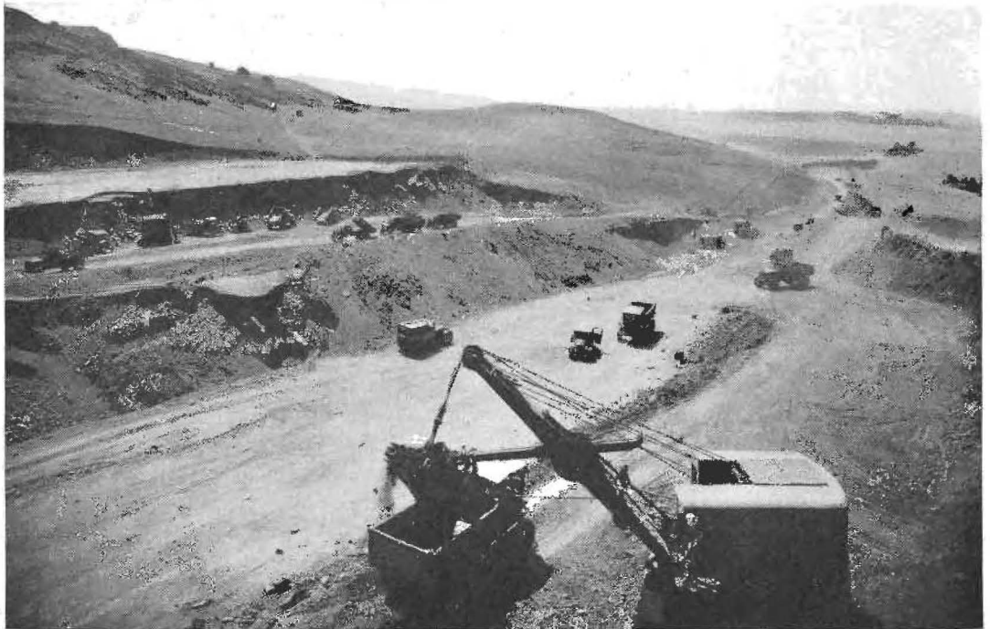
THE "BIG CUT" of the American Canyon cut-off project is the scene of busy operations to prevent further slides of top soil underlain by blue clay that lies in planes at abrupt angles. Power shovels and trucks are at work making broad terraces and removing material above the sliding planes back far enough to prevent further movement into the roadway.
