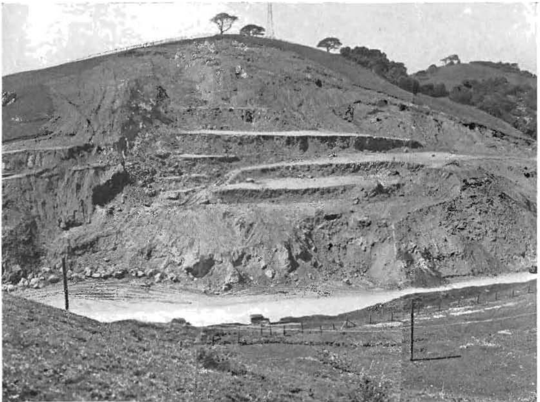
GIANT BENCHES WERE CUT for the removal of the slide material but the movements destroyed them almost as soon as they were graded. A total of 200,000 cubic yards of material was moved and the highway kept open at all times. Height of slide can be judged by comparison with size of the automobile on the highway in foreground.
