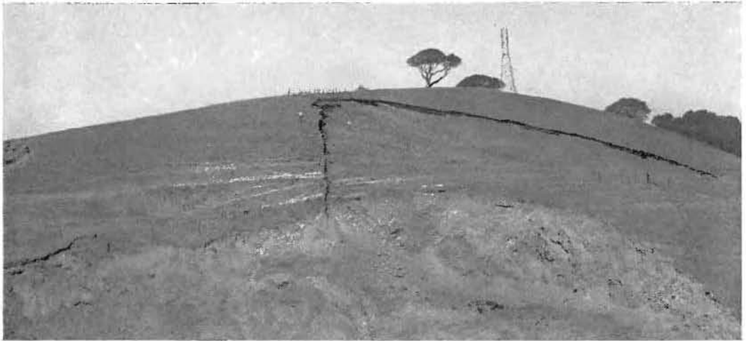
AN OMINOUS CRACK APPEARED after a rain period in a low spur of Mt. Tamalpais in Marin County and a great mass began moving down upon the highway cut.
