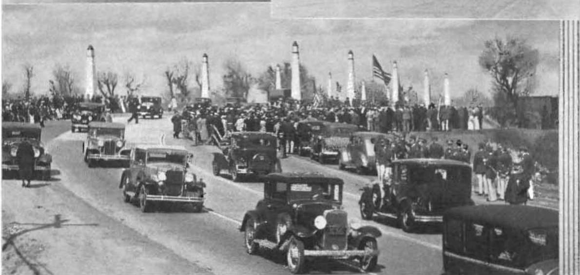
AMERICAN RIVER BRIDGE at Sacramento as transformed by the State Department of Public Works from a narrow, traffic bottleneck structure is pictured at top in photo by Hansaker of Bee from Barker-Witney Flying Service plane. White roadway area on upstream side indicates part added by widening operation and inset shows work under construction. Center photos show the old two-lane roadway and 65 foot radius curve approach on 8\frac{1}{2} per cent grade compared with the new 600 foot radius curve approach and 3 per cent grade. Bottom scene shows crowds gathering for the dedication ceremonies on March 24th, when Governor Merriam formally opened the reconstructed bridge to traffic.
