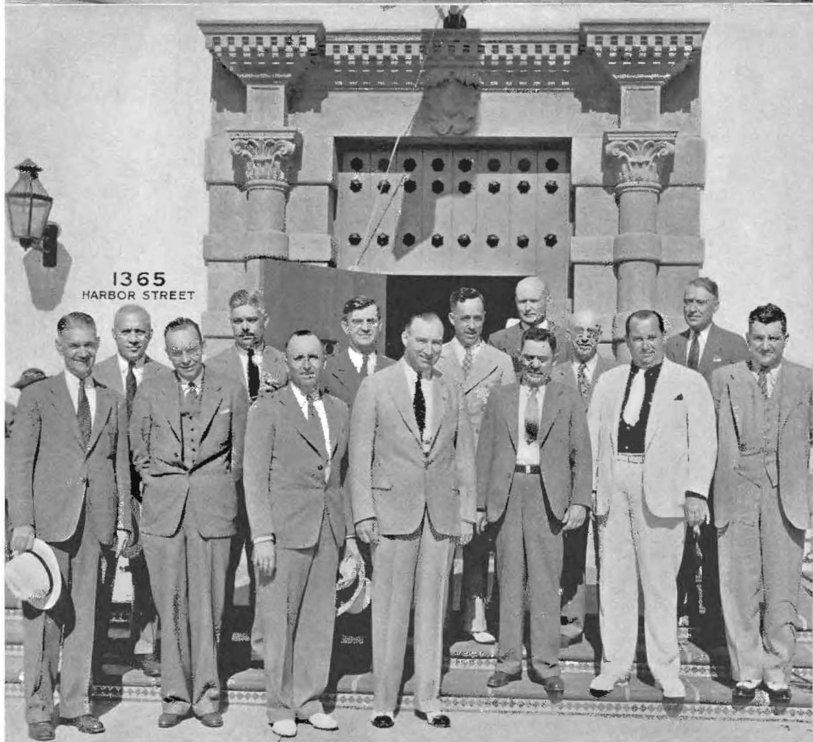
DEDICATION SCENES AT SAN DIEGO. At top, the new office building of District XI taken during dedication exercises just before the flag raising. Below in the official group, left to right, are State Construction Engineer C. S. Pope; H. S. Comly; President Jno. Fox, San Diego Chamber of Commerce; Acting Bridge Engineer F. W. Panhorst; Chairman F. G. Forward, Chamber of Commerce; J. F. Craemer, Assistant Director and Earl Lee Kelly, Director of Public Works; Principal Assistant Engineer J. G. Standley; District Engineer E. E. Wallace; H. A. Hopkins, Chairman, C. D. Hamilton, member, and Julien Roussel, secretary, of Highway Commission; C. C. Carleton, Chief Contracts and Rights of Way and Edward Neron, Deputy Director of Public Works.
