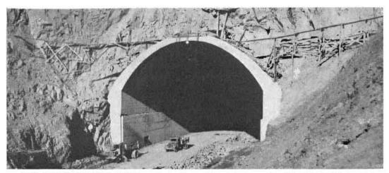
BAY BRIDGE TUNNEL BORE on Yerba Buena Island just completed is 76 feet wide by 58 feet high making it the largest bore tunnel in the world. Note size compared with trucks.
