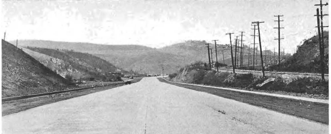
ALONG THE RAMONA "AIRLINE" HIGHWAY between Monterey Park and Los Angeles. The top view shows a section of the roadway on the grade separation where the new highway crosses Coyote Pass road near Monterey Park. Traffic going southwesterly into Coyote Pass is diverted and passed under the new highway by the road at the left of the picture and thus avoids a right hand turn. The center picture is a view of the long, wide straightaway approaching the concrete bridge that carries Eastern Avenue over the new highway and the Pacific Electric tracks. At bottom is a typical section paralleling the railroad showing the 40-foot pavement, wide oiled shoulders and curbing of this 6-mile stretch of high standard arterial without a grade crossing over which more than 20,000 cars will enter the Los Angeles Civic Center area.
