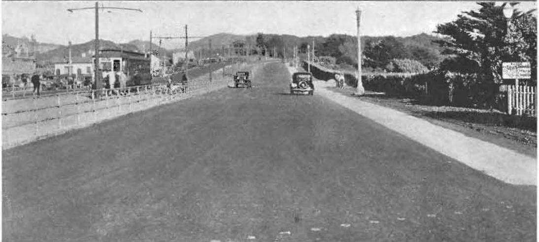
SLOAT BOULEVARD IMPROVEMENT: 1—At top, general view showing 135 foot right of way with one-way traffic on either side of trolley tracks in the center. 2—North side of highway at point opposite Fleishhacker Zoo and pool showing subway entrance to Municipal Beach. 3—South side of Sloat Boulevard Improvement at Beach Subway opposite entrance to Fleishhacker Pool.
