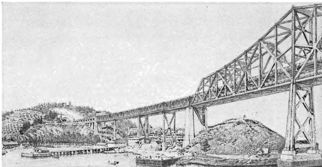
AN IMPRESSIVE PREVIEW of a section of the San Francisco-Oakland Bay Bridge just east of Yerba Buena Island, to be built during the first half of 1935, is presented in this drawing by Artist Nusé. A concrete viaduct extends from the tunnel mouth to a large concrete pier YB-1. Steel truss spans connect this pier with the huge concrete Anchor Pier E-1, that holds the anchor arm for the heavy cantilever span that will extend easterly from Pier E-2 shown at extreme right of picture.
