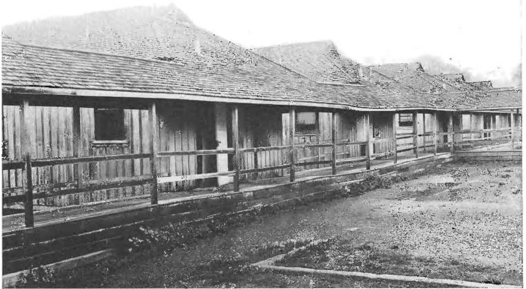
INSANITARY DILAPIDATED WOODEN SHACKS , known as the Dozier cottages, built in 1907 as temporary structures at Napa Hospital, still house 386 women mental patients, including tuberculosis cases.
