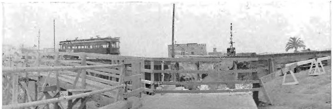
TEMPORARY TRESTLES for pedestrians and trolley cars are provided for the traffic on Ocean Avenue and to numerous beach resorts, especially heavy on weekends and holidays.
