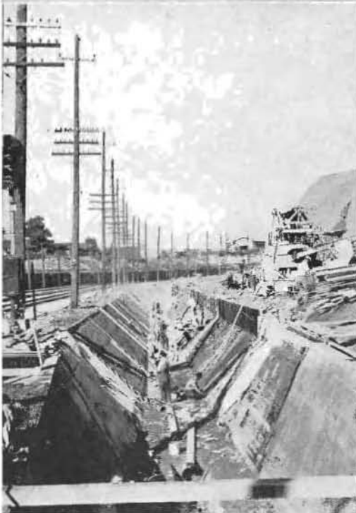
RAMONA BOULEVARD UNIT of the Los Angeles-Pomona airline arterial, presented some difficult construction between State Street and Mission Road, restricted for most of the distance between the railroad, a natural drainage channel and high bluffs, and passing under bridges carrying intersecting highways. A gunnite lined canal was constructed for the drainage channel.
