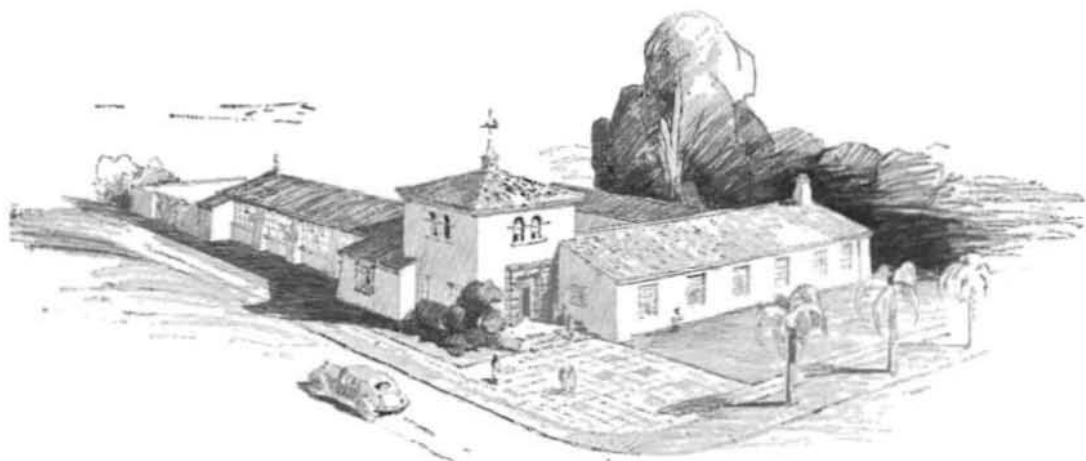
EARLY SPANISH in its architectural style, the new district office building of the Division of Highways in San Diego is of concrete construction, 115 feet long by 116 feet wide with a two story corner tower. Designed by the Division of Architecture of the State Department of Public Works.
