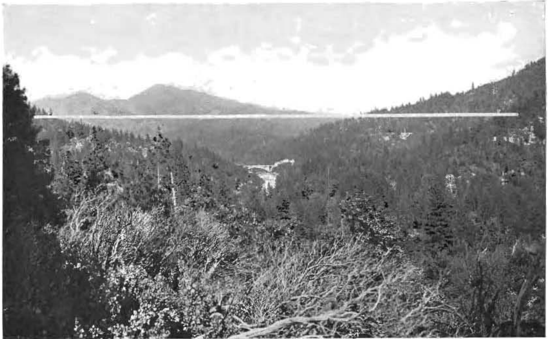
NEW BRIDGE SITE across the Pit River for the proposed joint highway and railroad bridge made necessary by the Kennett Dam project is indicated by the white line, 325 feet higher than present bridge shown in background.
