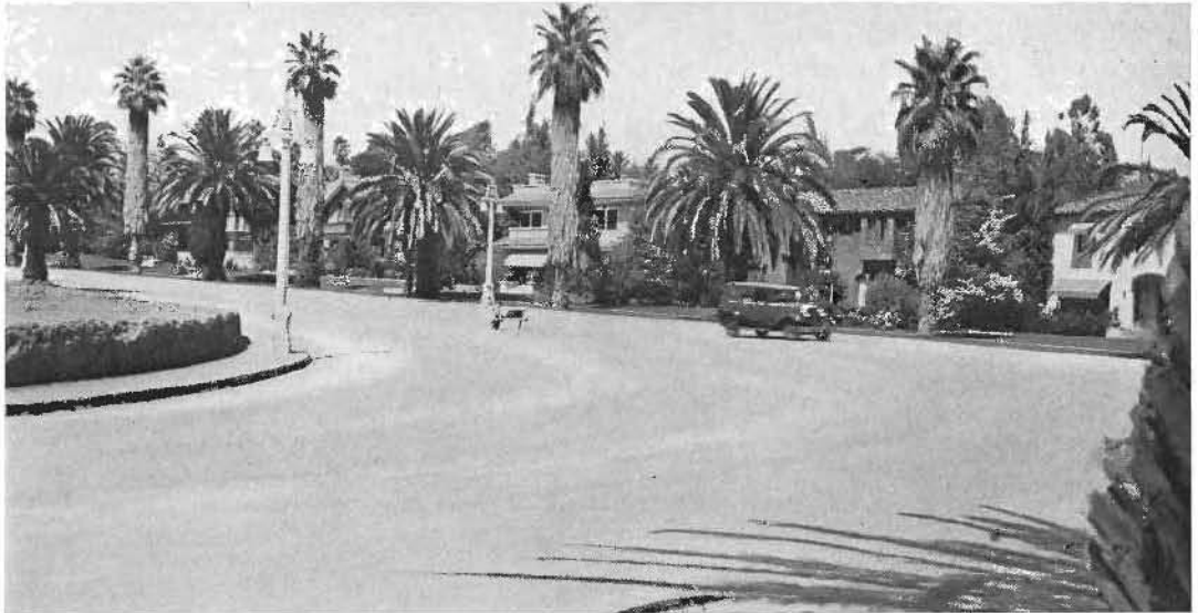
WEST ENTRANCE TO RIVERSIDE as realigned eliminating right angle turn, graded and paved with $12,769 of gas tax funds and $10,000 from State Cooperative fund.
