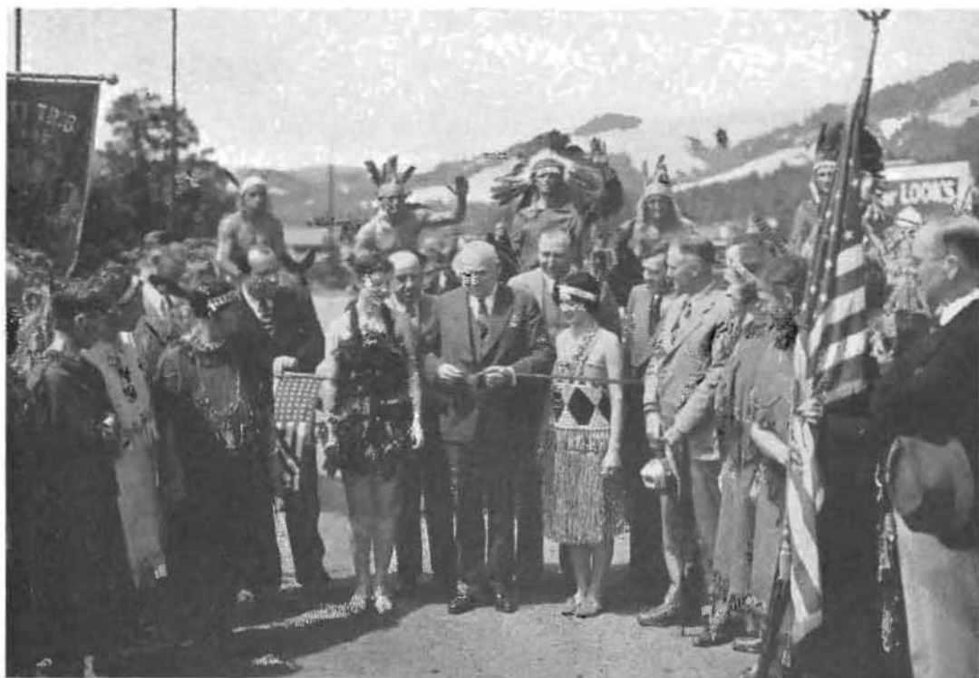
PICTURESQUE CEREMONY marked the ribbon-cutting scene at the dedication of the Benbow-Garberville unit of the Redwood Highway relocation project. Left to right, the State officials in the group are: Senator H. A. Perry; Highway Commission Secretary Julien D. Roussel; Commissioner T. A. Reardon; Governor Merriam; Director of Public Works Earl Lee Kelly; Assistant Director Justus F. Craemer; Commissioner Ray Ingels.
