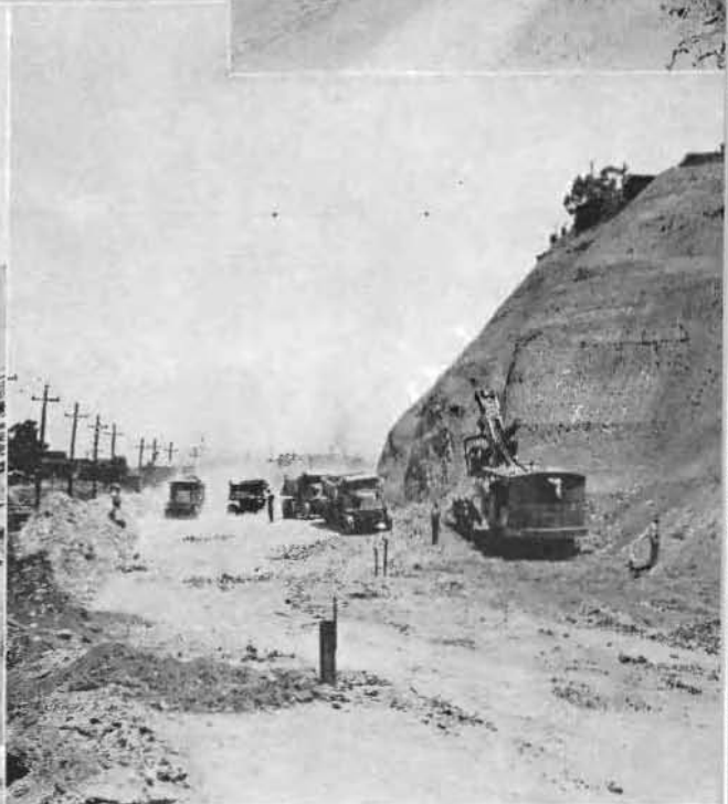
RAMONA BOULEVARD UNIT of the Los Angeles-Pomona airline arterial, presented some difficult construction between State Street and Mission Road, restricted for most of the distance between the railroad, a natural drainage channel and high bluffs, and passing under bridges carrying intersecting highways. A gunnite lined canal was constructed for the drainage channel.
