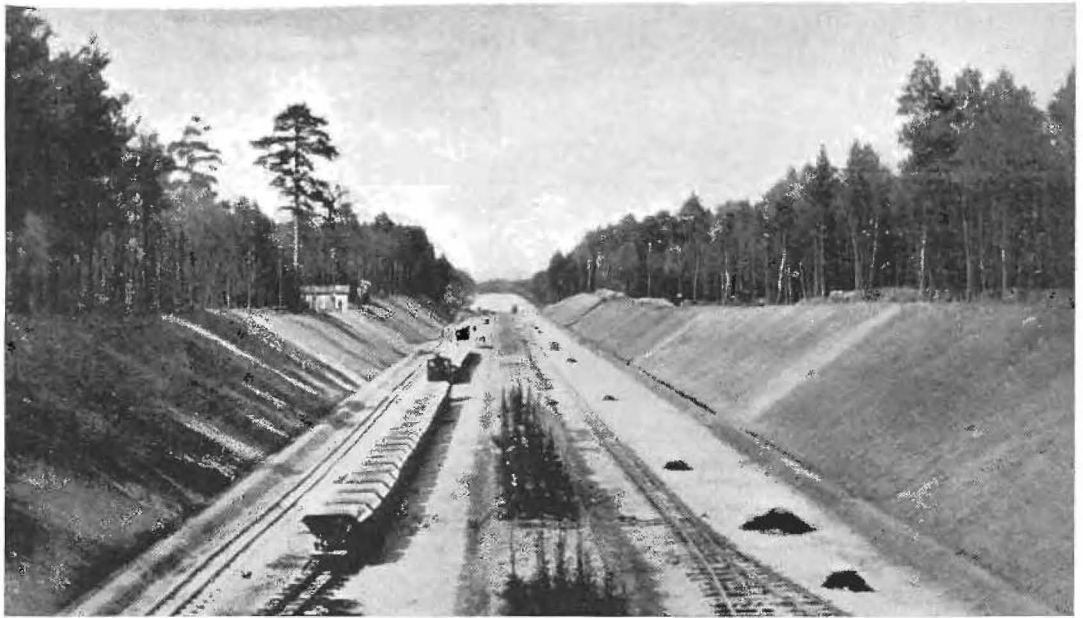
GERMAN EXPRESS HIGHWAY under construction. This typical section provides for a center lawn strip 15 feet wide, with a pavement 25 feet wide, consisting of two traffic lanes on either side bordered by shoulders. Note the planting of trees and shrubbery on center strip.
