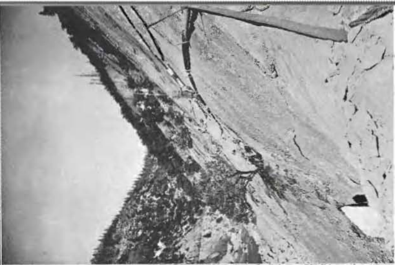
GREAT GRANITE DOMES of Feather River Canyon are being blasted and tunneled by highway engineers. The top picture shows the end of grading at Arch Rock where drilling operations begin. The upper line across the rock is a 4-inch airline for supplying the jackhammers. The other lines provide footholds for the men. Lower left photo shows 9 by 14 foot heading of tunnel No. 1. Outline for the completed tunnel is shown on face of portal. At lower right, men are loading drill holes on steep bare slope.
