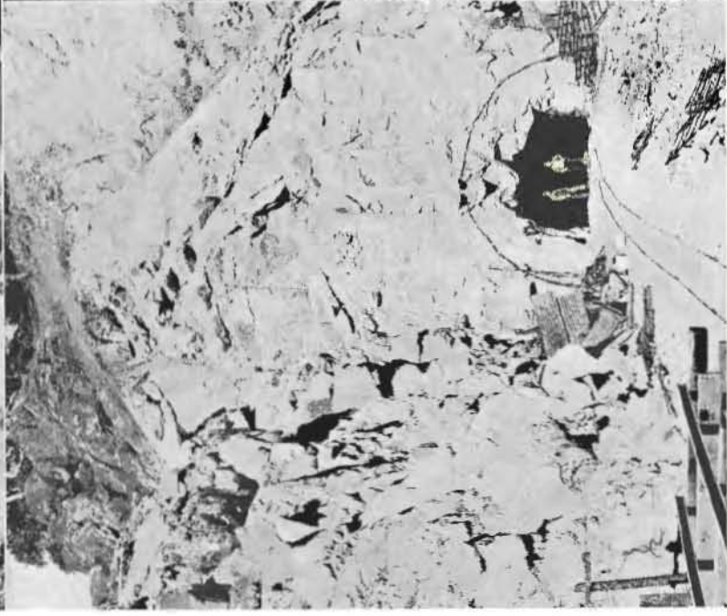
GREAT GRANITE DOMES of Feather River Canyon are being blasted and tunneled by highway engineers. The top picture shows the end of grading at Arch Rock where drilling operations begin. The upper line across the rock is a 4-inch airline for supplying the jackhammers. The other lines provide footholds for the men. Lower left photo shows 9 by 14 foot heading of tunnel No. 1. Outline for the completed tunnel is shown on face of portal. At lower right, men are loading drill holes on steep bare slope.
