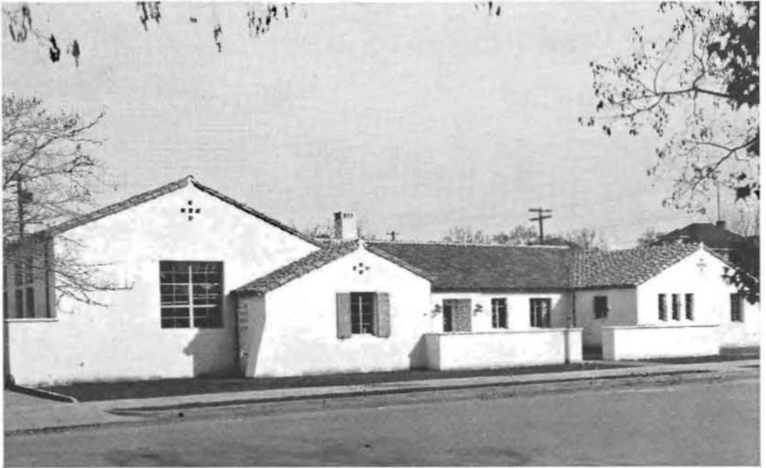
NEW DISTRICT HEADQUARTERS BUILDING in Stockton is a one story reinforced concrete structure 121 x 82 feet located at Center and Rose Streets. It has 11 office rooms in addition to a public lobby, information room, stock room and basement.
