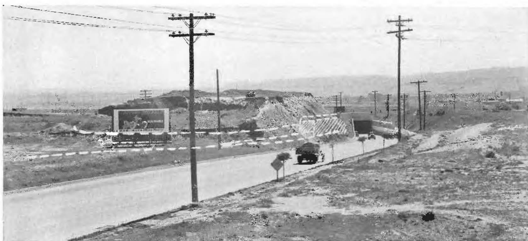
TRAFFIC DEMANDS MORE ROOM in the South San Francisco underpass on Bayshore Highway. Dotted lines on photo of Southern approach show proposed widening operation on structure, hillside and roadway.
