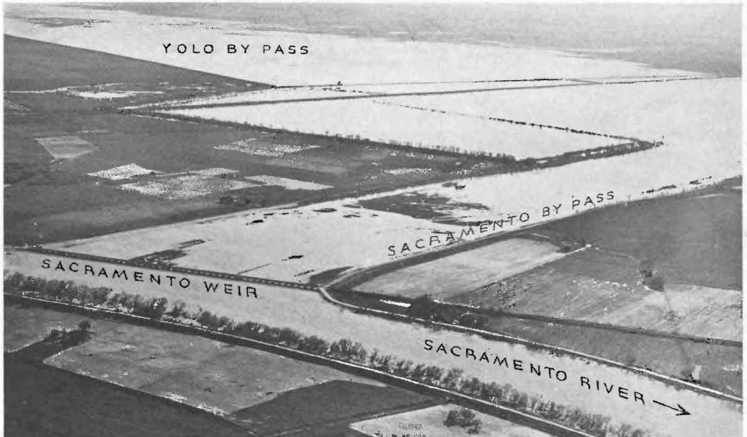
BY-PASS AND WEIR IN OPERATION —Aerial view of normally dry land in the vicinity of Sacramento on which excess waters of the Sacramento River are being distributed and carried off through the Sacramento Weir, Sacramento by-pass and Yolo by-pass units of the Sacramento Flood control Project.
