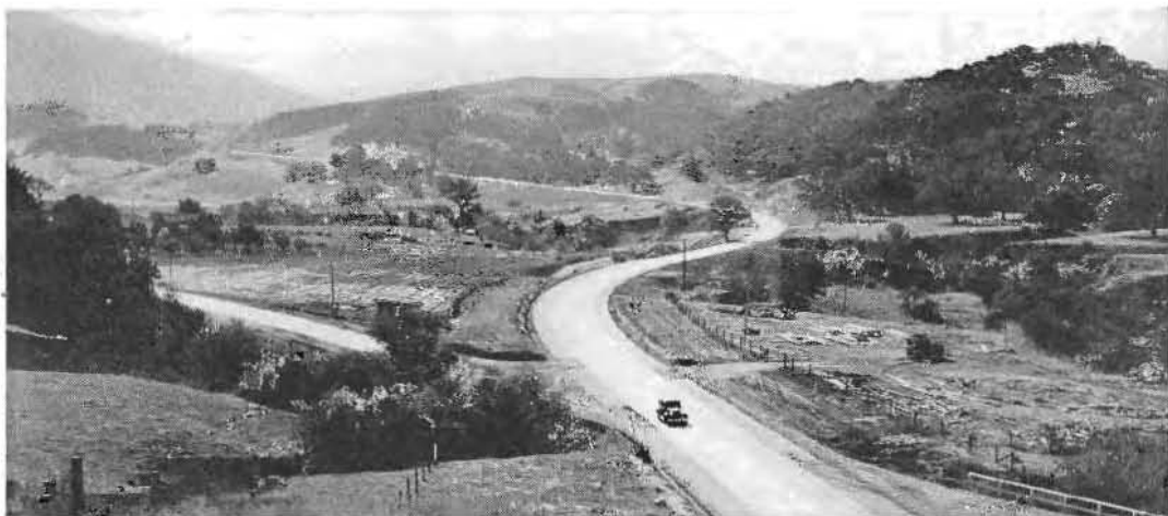
NEW ROUTE climbs through the hills on an easy 6 per cent maximum grade made possible by deep cuts representing 670,000 cubic yards of excavation and shortening the distance by nearly a mile.
