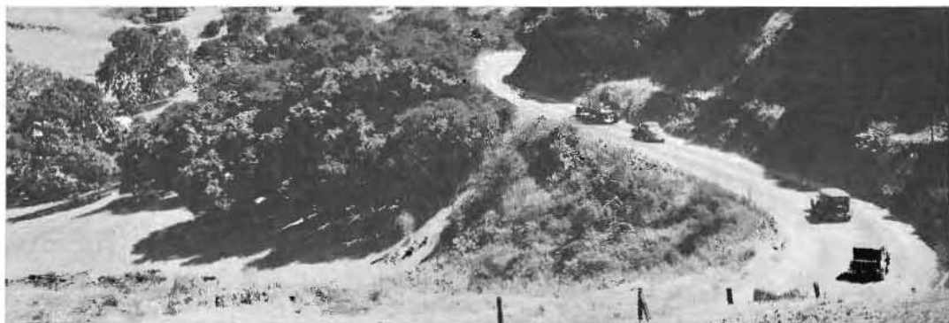
OLD ROUTE abounded in hairpin turns such as the two shown in the above picture taken before the improvement when traffic was compelled to loiter along behind heavily laden trucks.
