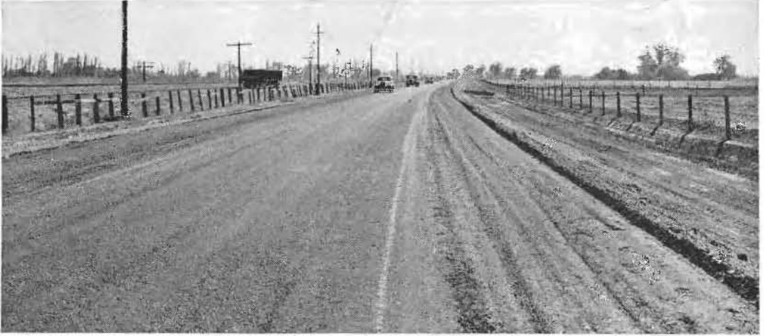
STRAIGHT AND WIDE runs the new highway for 4.54 miles between Newman and Crows Landing on State Route No. 41, cutting out many dangerous curves on the narrow old county route.
