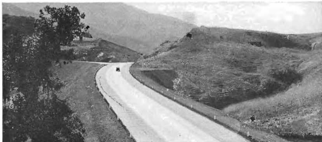
NOJOQUI GRADE through Gaviota Pass in Santa Barbara County has been transformed from a narrow, tortuous series of 44 sharp curves to a wide highway with only 11 long radius curves.
