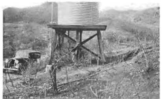
WATER TANK where men waged desperate fight with flames to save only water supply.
