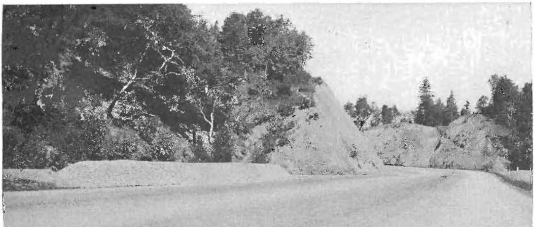
Los Gatos-Santa Cruz highway (State Route 5) paved with 40-foot bituminous macadam.
