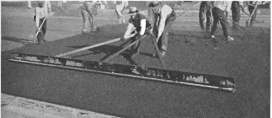
HAND FINISHING warped intersection pavement at Fresno street with 14-foot pole push float.
