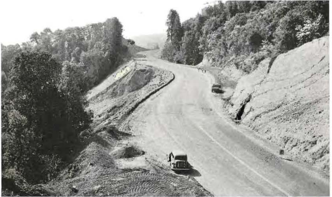
BIG FILL on the Los Gatos-Santa Cruz highway (State Route No. 5) showing where slide occurred threatening to entirely destroy the completed roadway last Spring
