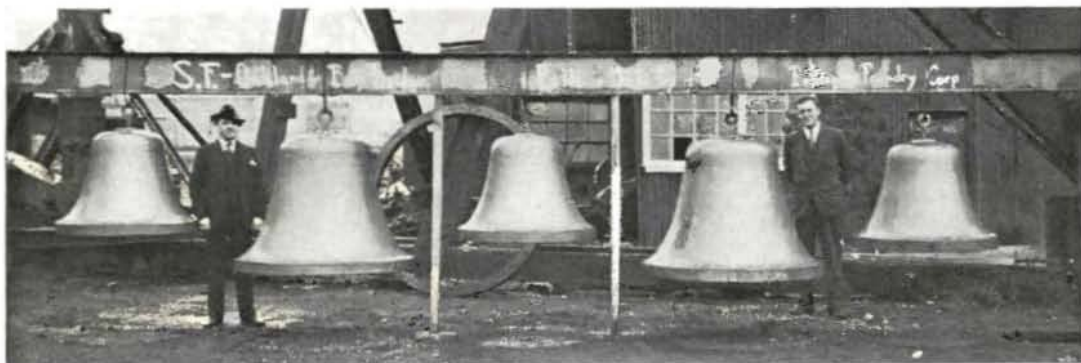
FIVE BIG BELLS that will ring out across the bay in fog and storm to warn skippers of the location of the Bay Bridge channel piers.
