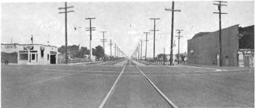
PEAK HOUR PERILS confront motorists at Graham Station on State Route 174 where Pacific Electric Interurban trains cross Firestone Boulevard in Los Angeles. The danger will be eliminated by construction of a subway under the tracks.
