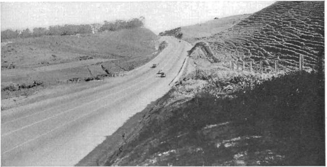
JUNIPERA SERRA HIGHWAY in San Mateo County with 40-foot pavement of asphalt concrete.
