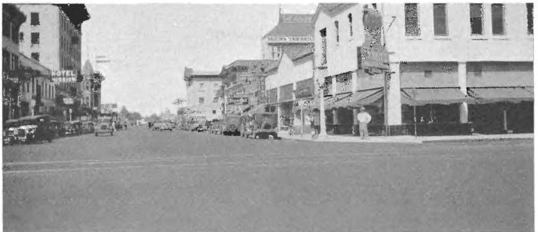
COMPLETED JOB of asphalt concrete pavement at intersection of Fresno street and Broadway.
