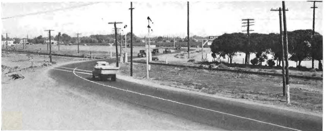
GRADE CROSSING on "S" curve at Delano on the Golden State highway. This bad situation is being corrected with a realignment of the highway and construction of an underpass.
