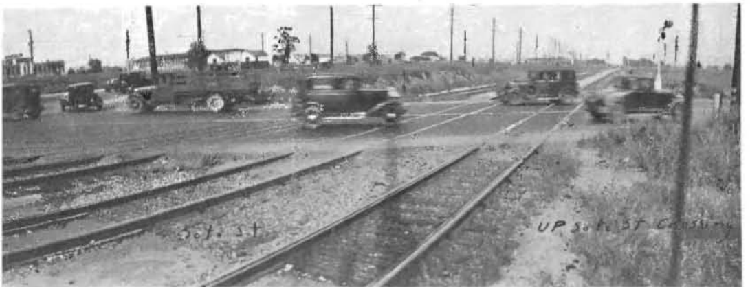
FOUR TRACK CROSSING of the Union Pacific's Main and Butte Street line on Soto Street in the city of Los Angeles. A subway will provide safety for vehicular traffic.
