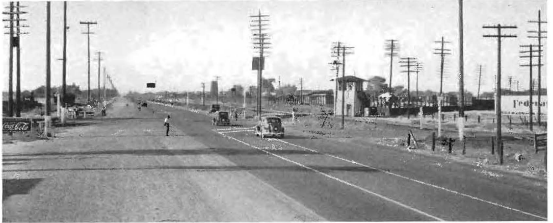
A DOUBLE DANGER is encountered at Calwa where the Santa Fe railroad crosses the Golden State highway and the Southern Pacific tracks at grade. An overhead structure will be provided for motor vehicles.
