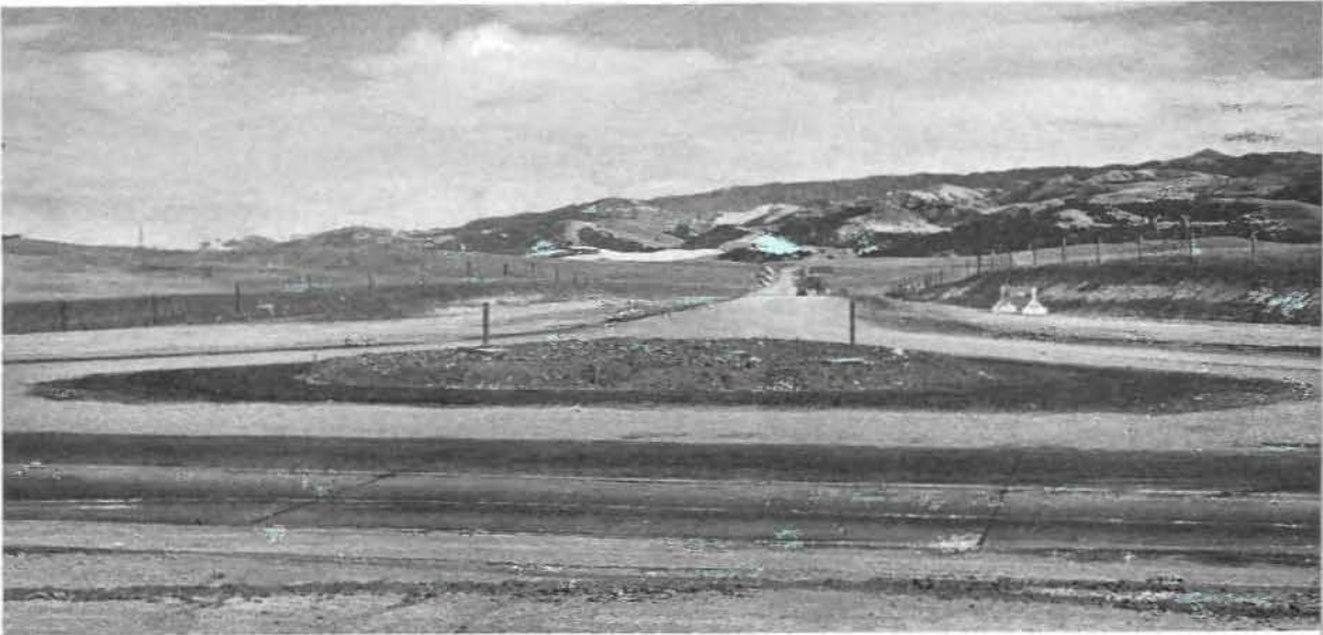
CROSS AND CAMPANILE will mark this intersection of the new road to the mission town of San Juan Bautista with the Prunedale cutoff.
