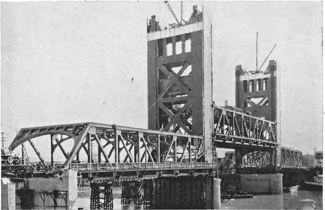
NEARING COMPLETION, the M Street bridge over the Sacramento River at the State capital is pictured with the 202-foot steel truss lift span in raised position still partially supported by false work.
