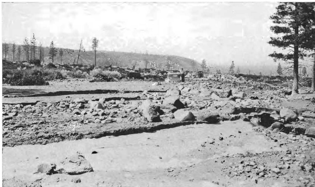
DEBRIS FROM SHASTA GLACIER flood waters covered State Highway 72 in storm of August 28 to a depth of four feet as shown in pictures on this page and page 29.
