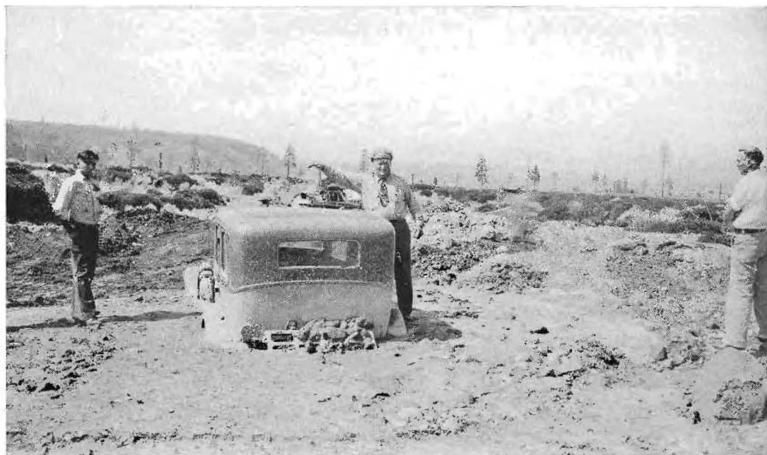
DEBRIS FROM SHASTA GLACIER flood waters covered State Highway 72 in storm of August 28 to a depth of four feet as shown in pictures on this page and page 29.
