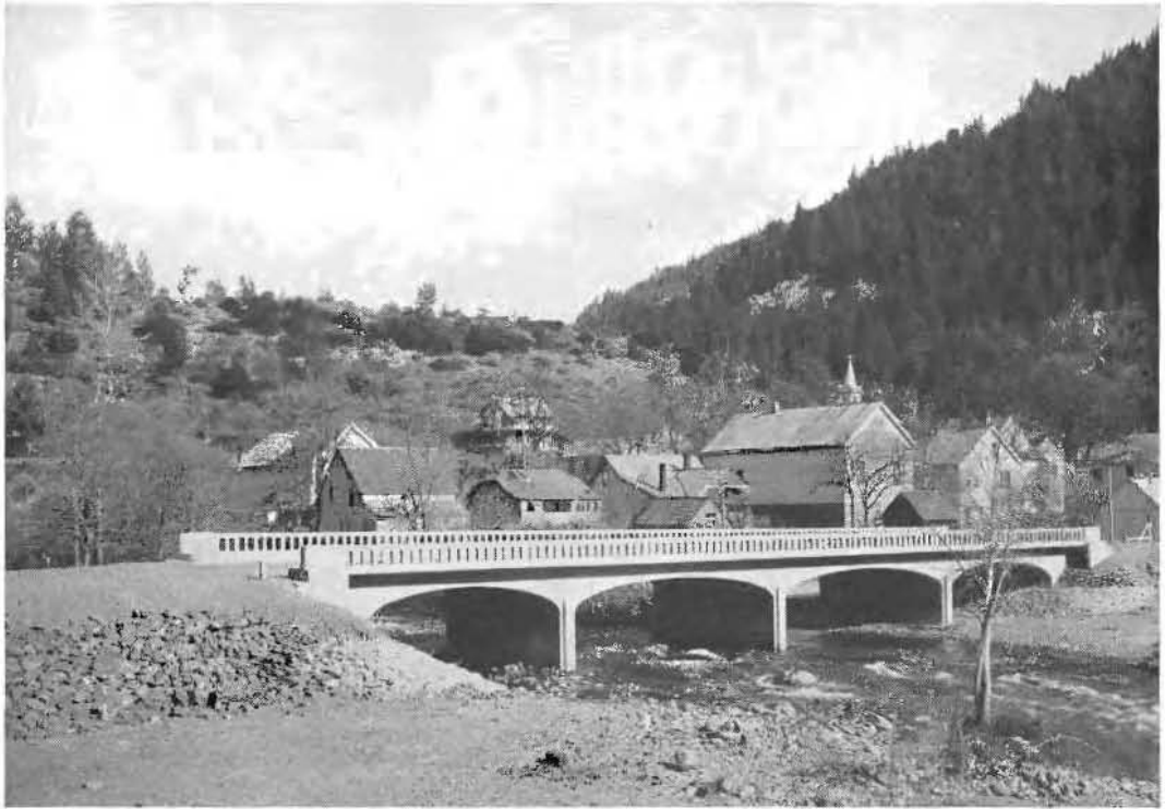
New reinforced concrete girder bridge on realigned State Highway across the North Fork of North Yuba River at Downieville.
