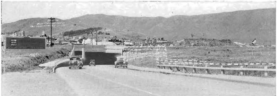
BEFORE WIDENING —Dotted lines show how additional space was provided for traffic and superstructure.
