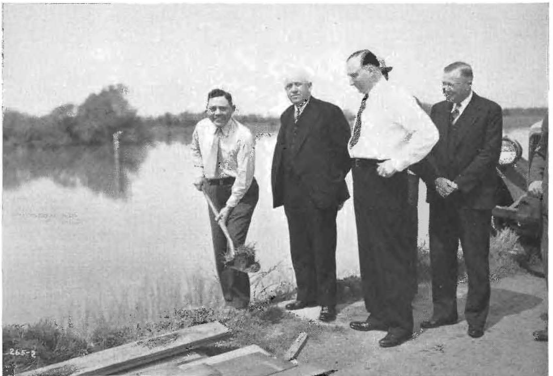
TURNING THE FIRST SHOVELFUL of earth in the groundbreaking ceremonies for the new drawbridge is Harry A. Hopkins, chairman of the California Highway Commission. Others are: Commissioner T. A. Reardon; Director of Public Works Earl Lee Kelly, who also did some shoveling, and District Engineer R. E. Pierce.
