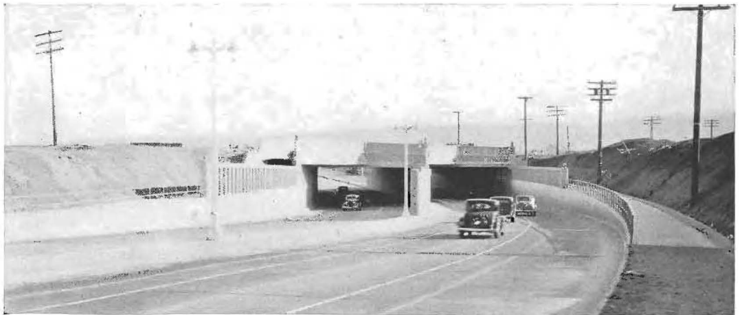
WIDENED TRAFFIC LANES separated by a curbing are shown in view of north side of underpass.
